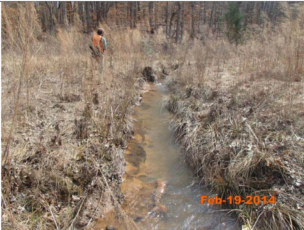
Reach 2 Sta. 309+50– Riffle Degradation
