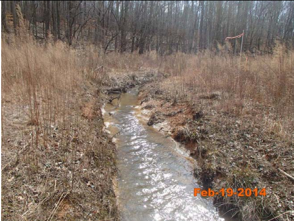
Reach 1 Sta. 305+50 – Riffle Degradation
