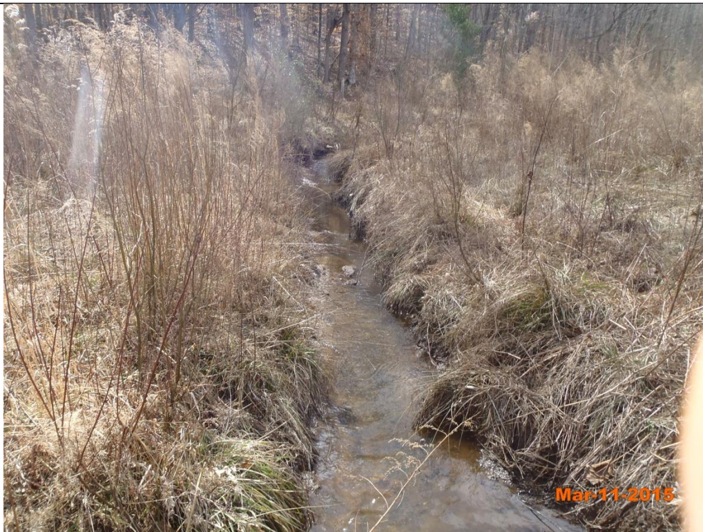
Reach 2 Sta. 309+50– Riffle Degradation
