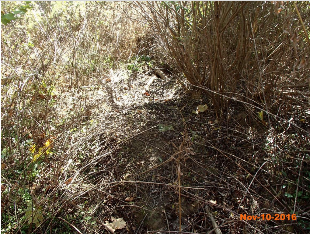
Reach 4 Sta. 101+50 – Channel Aggradation
