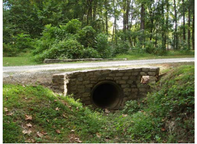
Photo 4. UT-2 crossing under gravel road
