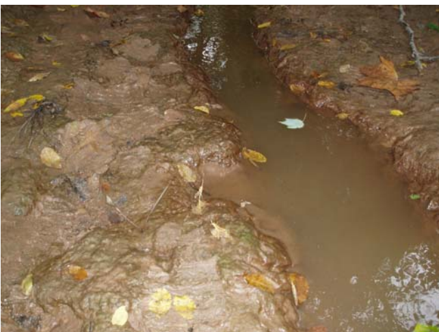
Photo 5. Hard-packed clay lining low flow channel
