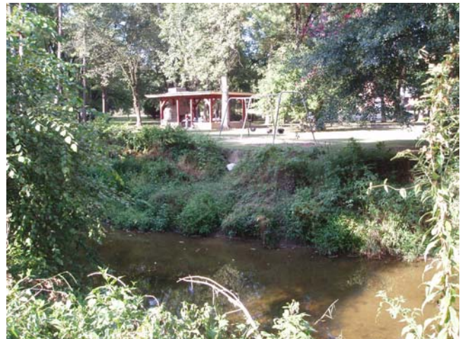
Photo 6. Eroding banks adjacent to park equipment
