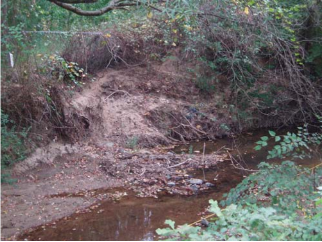
Photo 3. Eroding, sloughing banks in the upstream portion of the Project Reach
