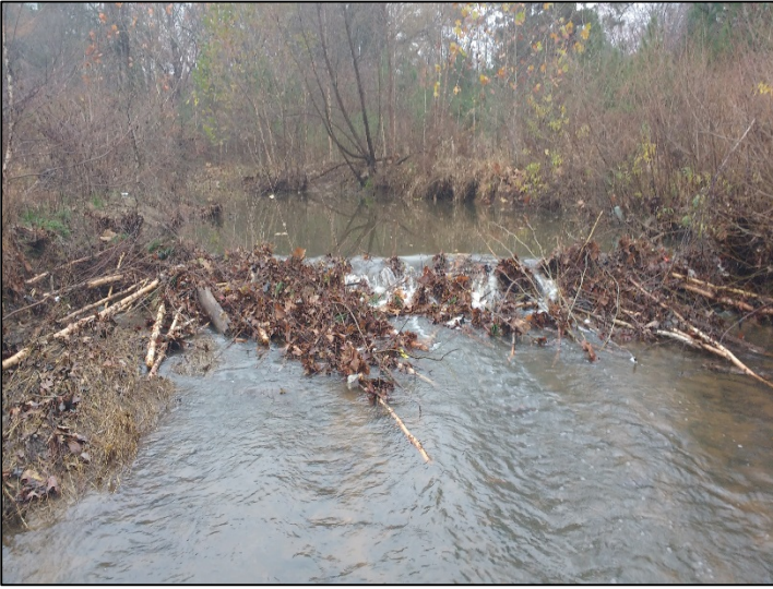
Beaver dam at Station 30 + 00. 12/2/2015
