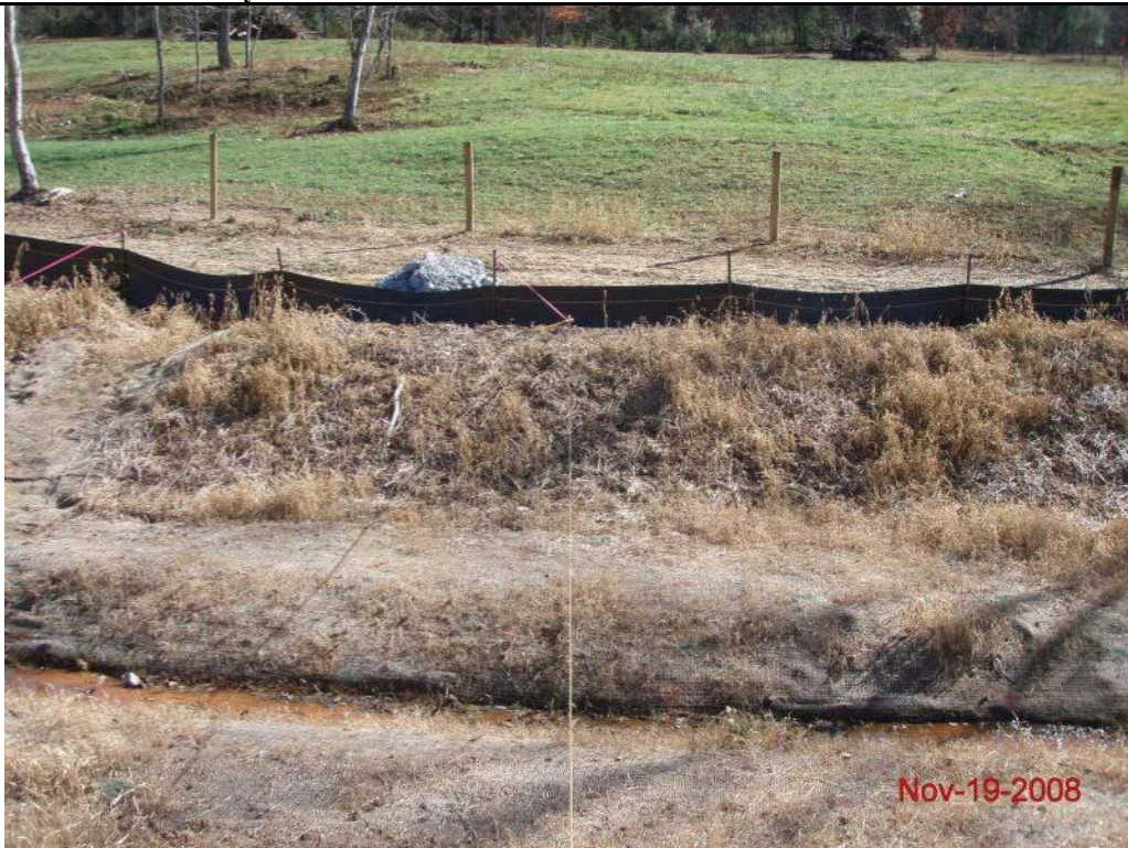
UT1 Upper – Cross Section 2 – Riffle Looking at Left Bank
