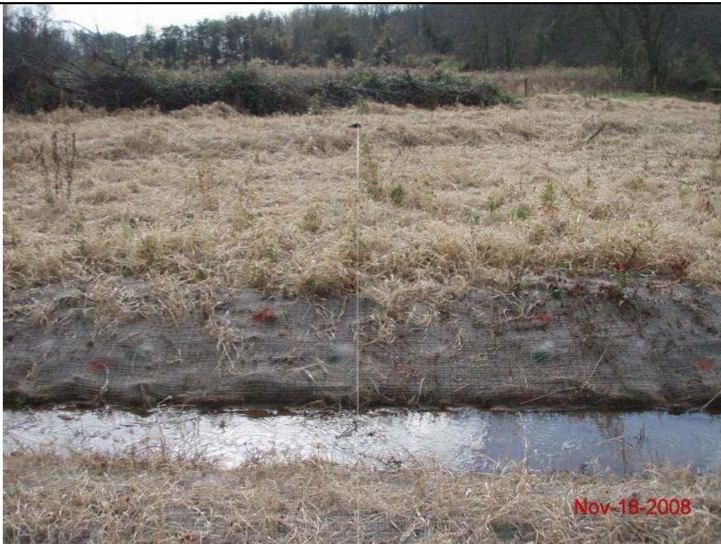
UT6 – Cross Section 3 – Riffle Looking at Right Bank
