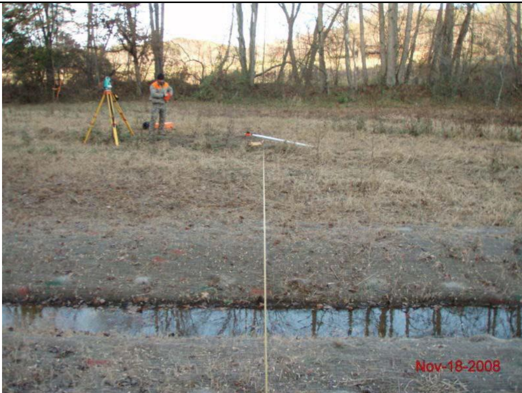
UT5 – Cross Section 2 – Riffle Looking at Right Bank
