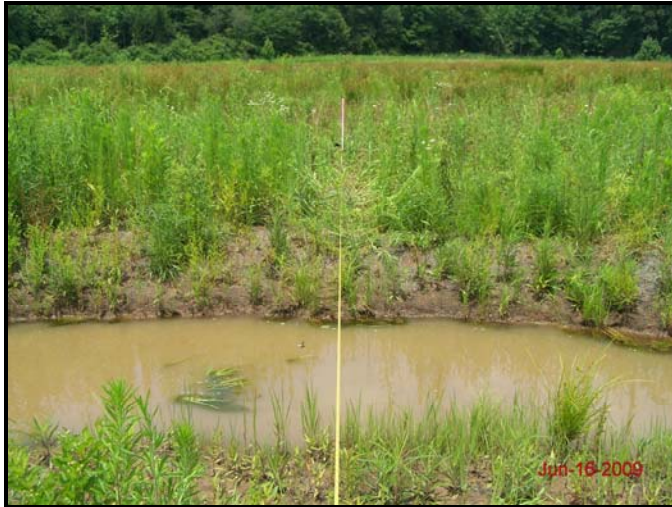
Looking at Left Bank
