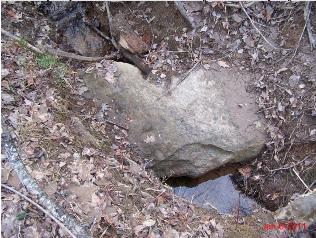
SPA9 UT5 Sta. 515+80 – Grade Control Degradation
