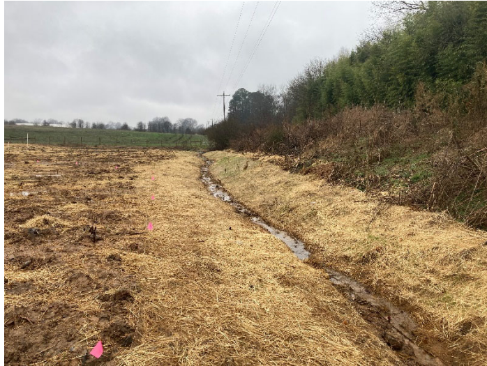
PP27 – Left floodplain ditch looking upstream (02/24/2022)
