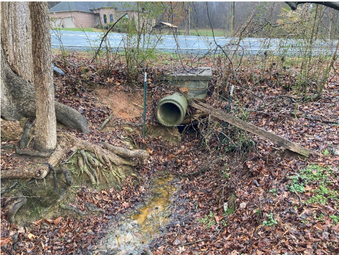
PP4 – UT1B looking upstream (02/24/2022)
