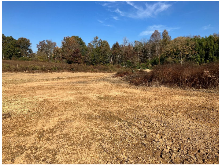
LFP OAK HILL CRK R4 – STA 121+00 NORTHWEST (10/24/2022)
