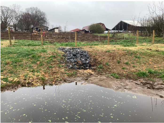
PP1.1 – BMP 1 looking north (02/24/2022)
