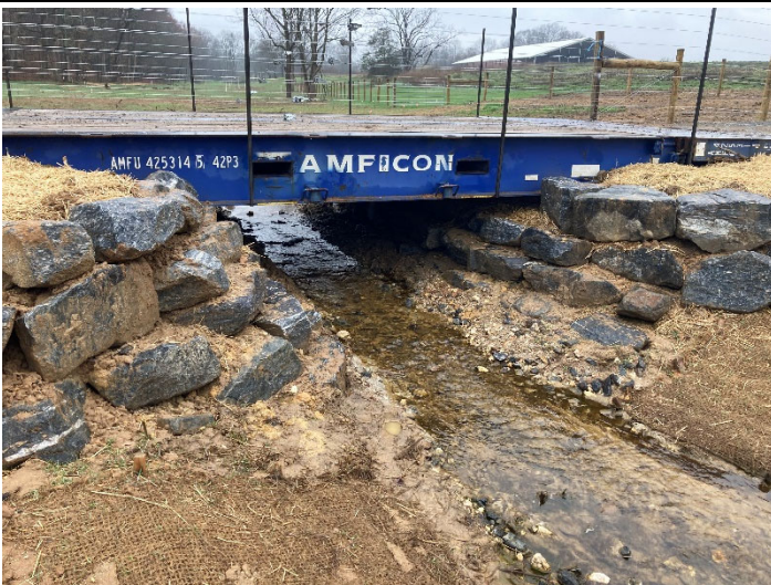
PP13 – UT1 R2 looking upstream (02/24/2022)
