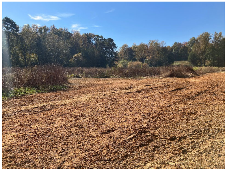
LFP OAK HILL CRK R3 – 111+98 SOUTHEAST (10/24/2022)
