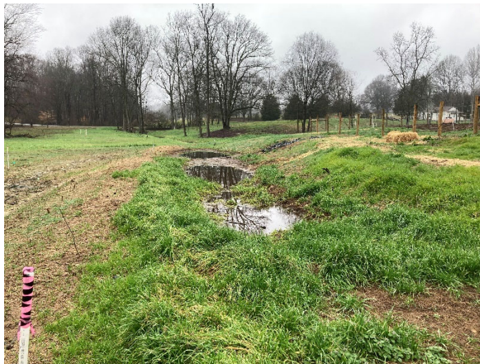
PP1.2 – BMP 1 looking west (02/24/2022)
