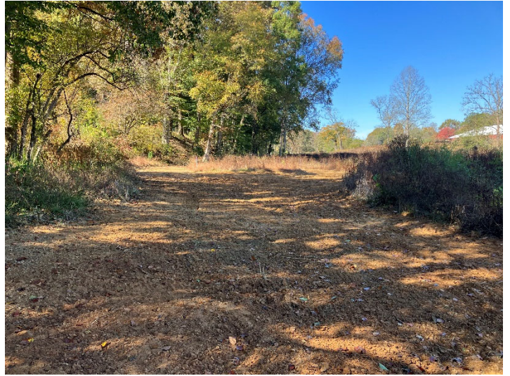
RFP UT1 R2 – STA 115+75 NORTHWEST (10/24/2022)
