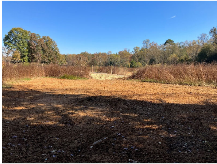
RFP UT1 R2 – STA 115+75 NORTHEAST (10/24/2022)
