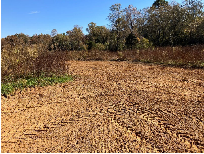
RFP UT2 – STA 219+00 SOUTHEAST (10/24/2022)
