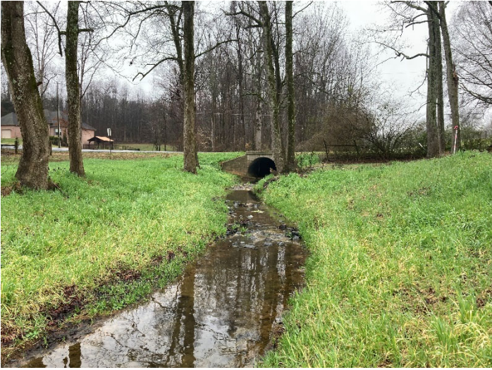
PP3 – UT1 R1 looking upstream (02/24/2022)
