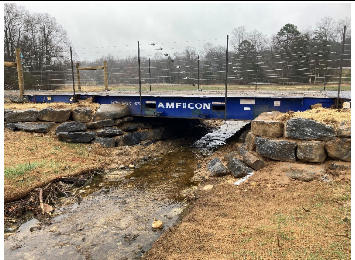
PP11 – UT1 R2 looking downstream (02/24/2022)
