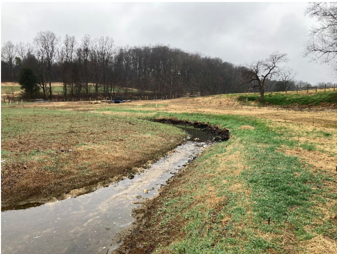
PP20 – UT1 R2 looking upstream (02/24/2022)
