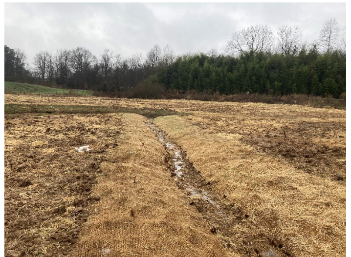
PP26 – Right floodplain ditch looking downstream (02/24/2022)
