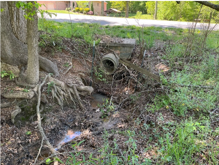
PP4 – UT1B looking upstream (04/24/2023)
