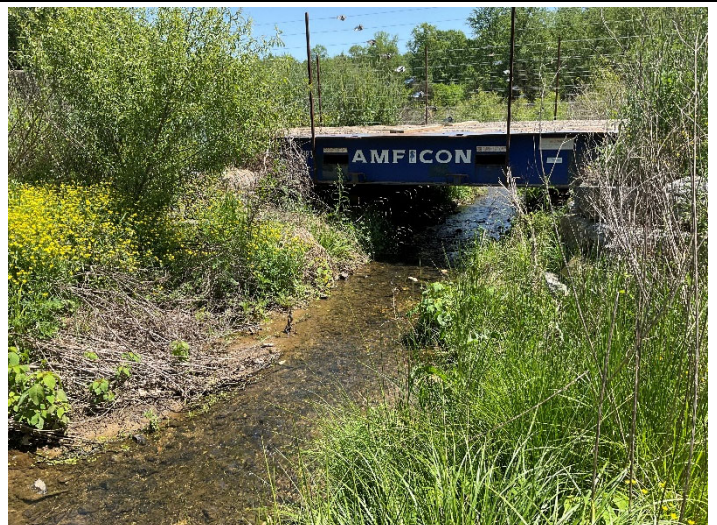
PP11 – UT1 R2 looking downstream (04/24/2023)
