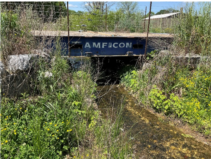
PP13 – UT1 R2 looking upstream (04/24/2023)
