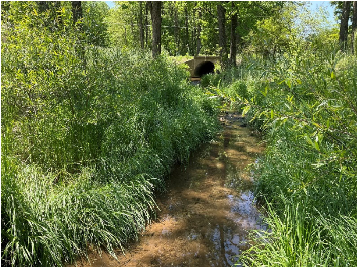
PP3 – UT1 R1 looking upstream (04/24/2023)
