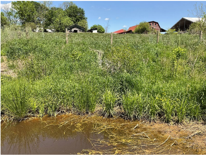
PP1.1 – BMP 1 looking north (04/24/2023)
