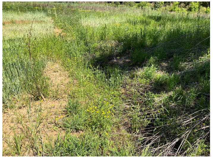
PP26 – Right floodplain ditch looking downstream (04/24/2023)
