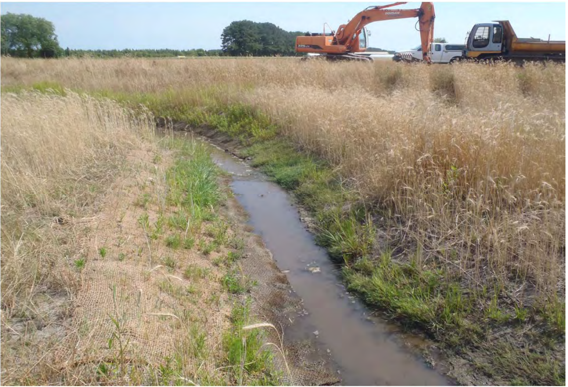
Sta. 35+24 Looking Downstream
