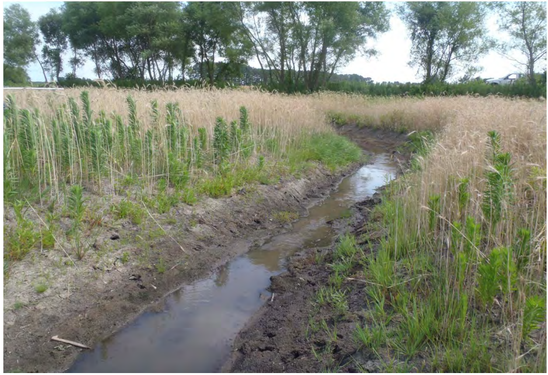
Sta. 28+46 Looking Downstream
