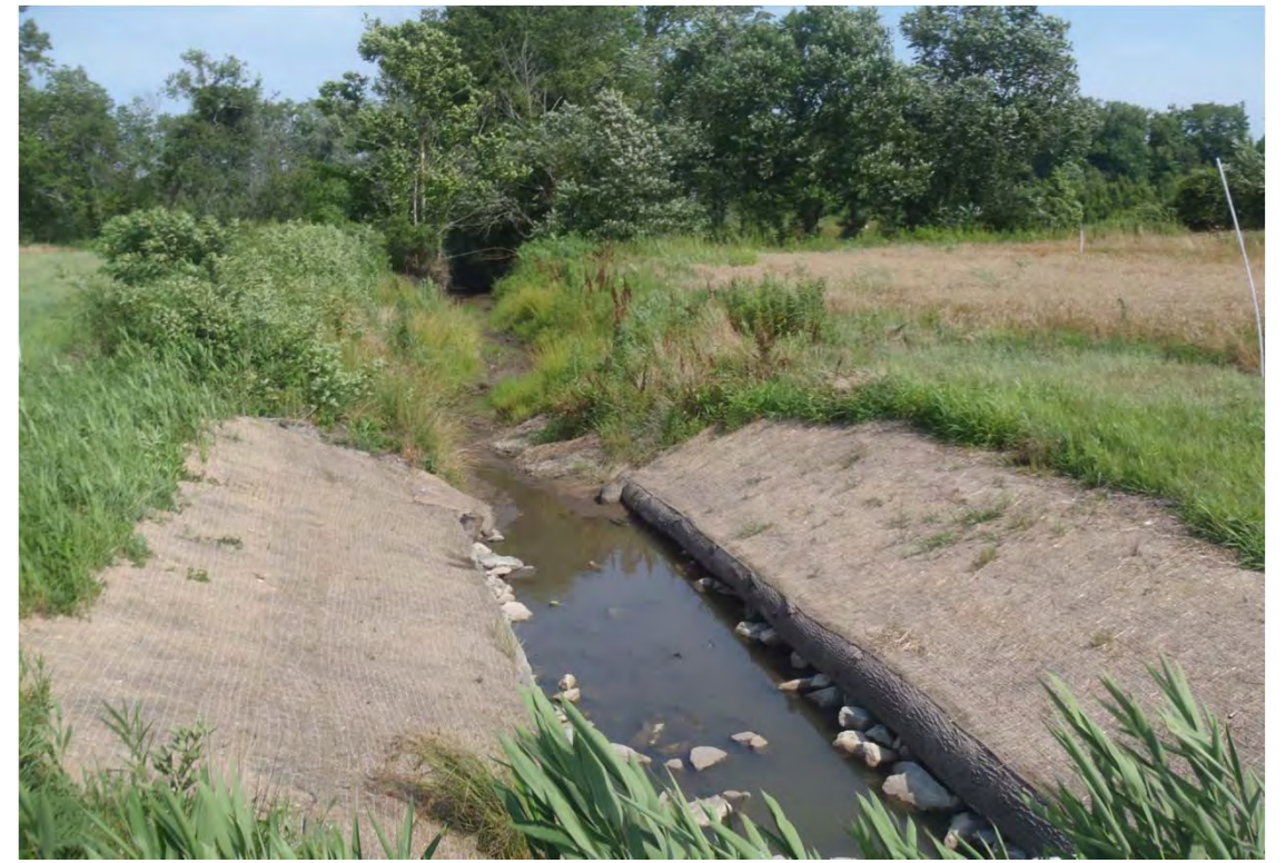
Sta. 38+71 Looking Downstream
