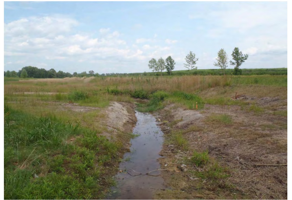
Sta. 0+75 Looking Downstream
