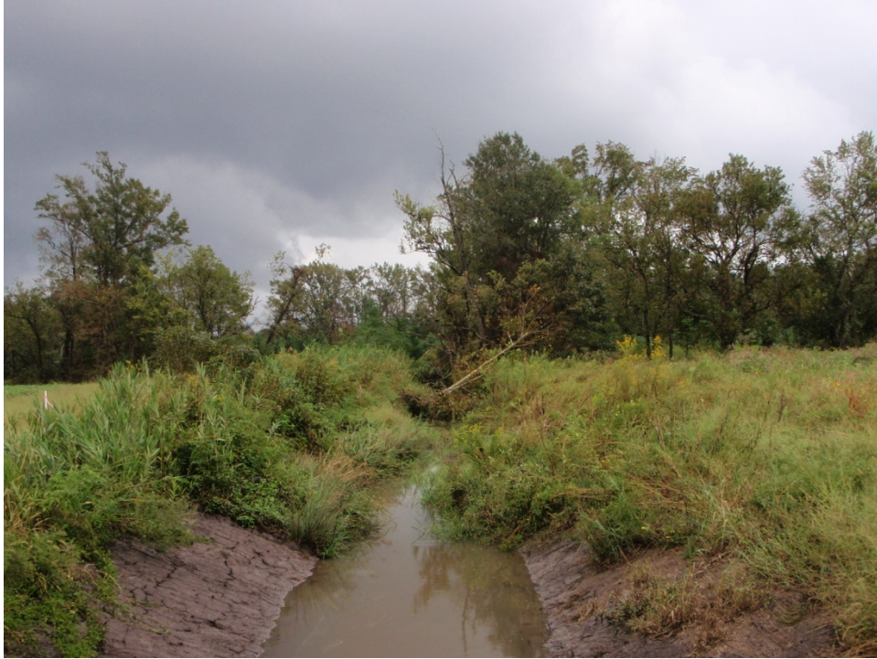
Photo Station S7 – Stream channel looking downstream at cross-section 7 Station 38+71 – Enhancement 2 (9/23/2011 Year 1)
