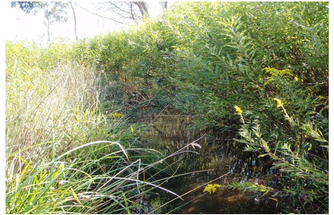
Sta. 32+71 Looking Downstream
