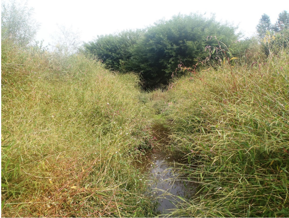
Photo Station S1 – Stream channel looking downstream at cross-section 1 Station 00+72 - Priority 2 (10/07/14 Year 4)
