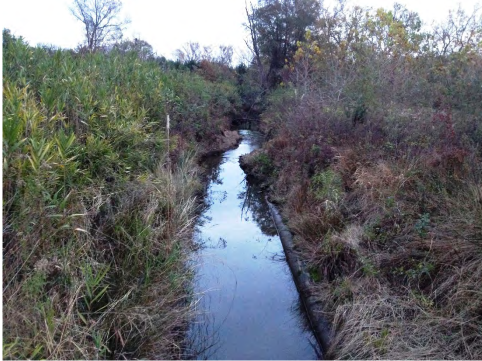
Photo Station S7 – Stream channel looking downstream at cross-section 7 Station 38+71 – Enhancement 2 (11/17/2015 Year 5)
