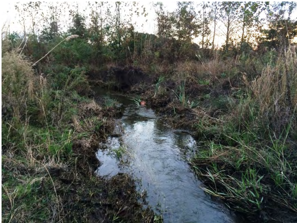
Photo Station S6 – Stream channel looking downstream at cross-section 6 Station 35+24 – Priority 2 (11/17/2015 Year 5)
