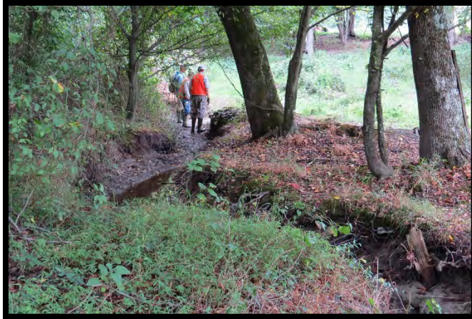
R4 looking downstream towards the bottom of the project limits. Note the lack of adequate riparian buffer along the right floodplain.
