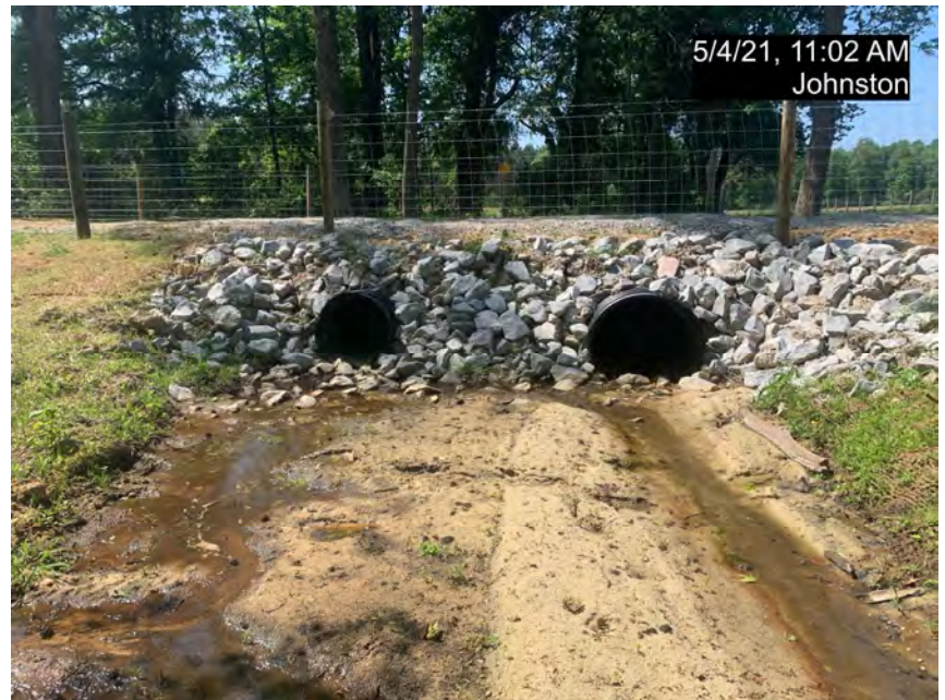
PS-2 – R2 Culvert Crossing, Downstream (MY-00)
