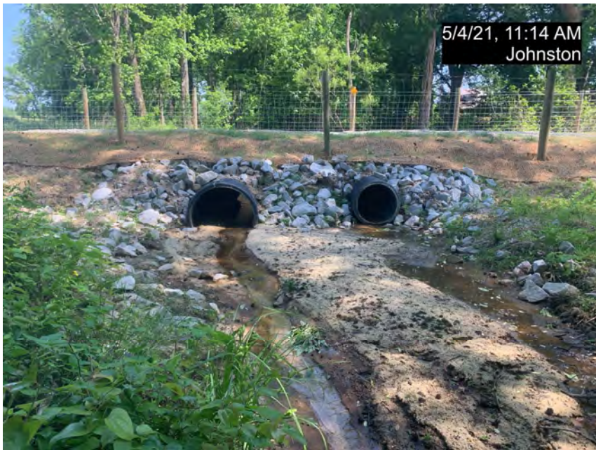
PS-2 – R2 Culvert Crossing, Upstream (MY-00)
