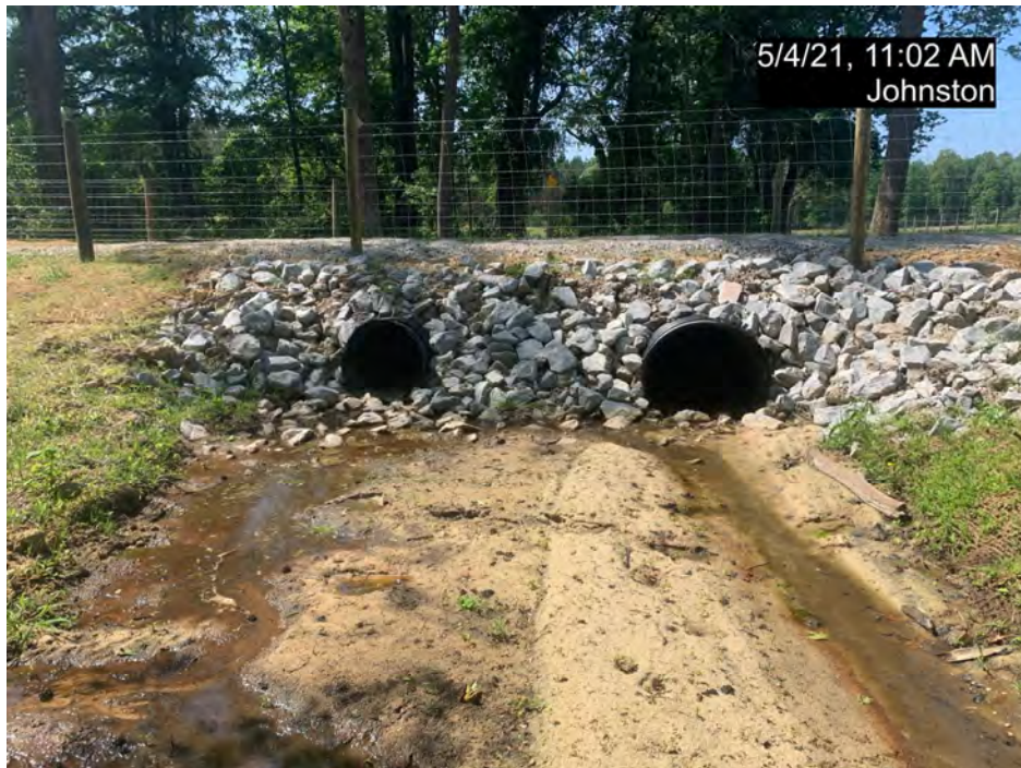
PS-2 - R2 Culvert Crossing, Downstream (MY-00)
