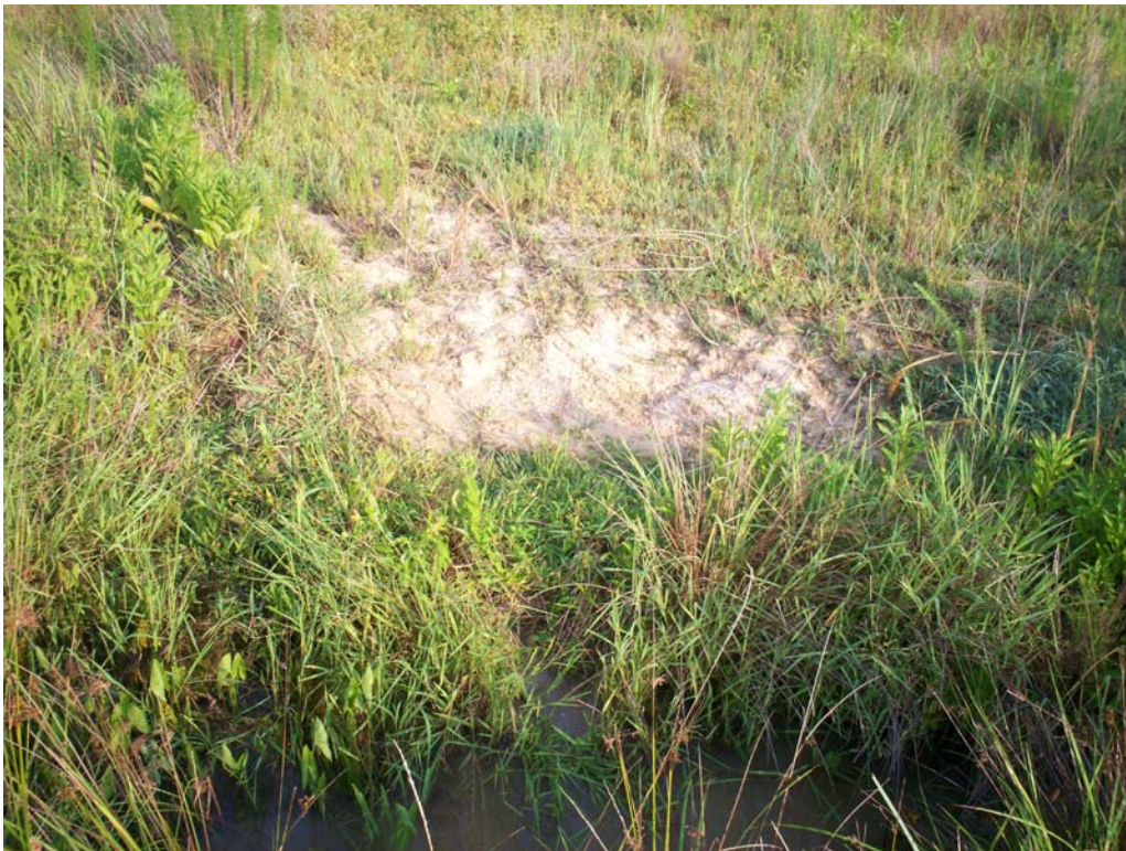
Photo 22. SPA 2. Right bank erosion due to sparse vegetation at STA 25+50.
