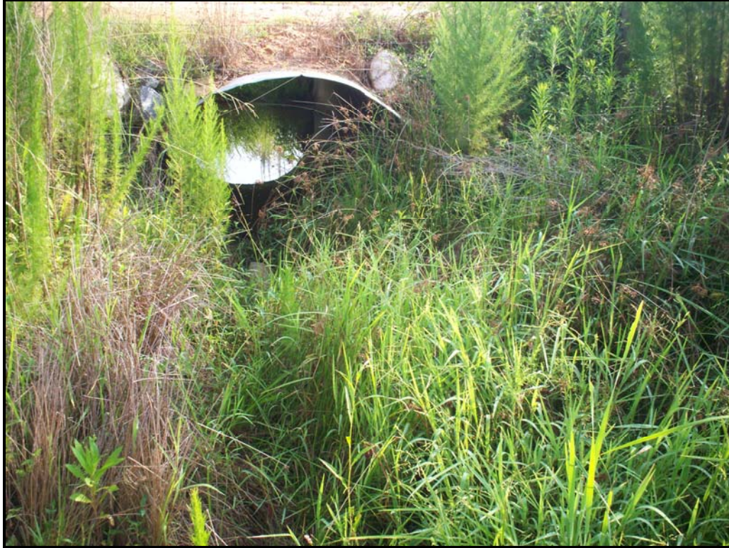
Photo 7. Culvert at STA 20+60 - looking upstream.
