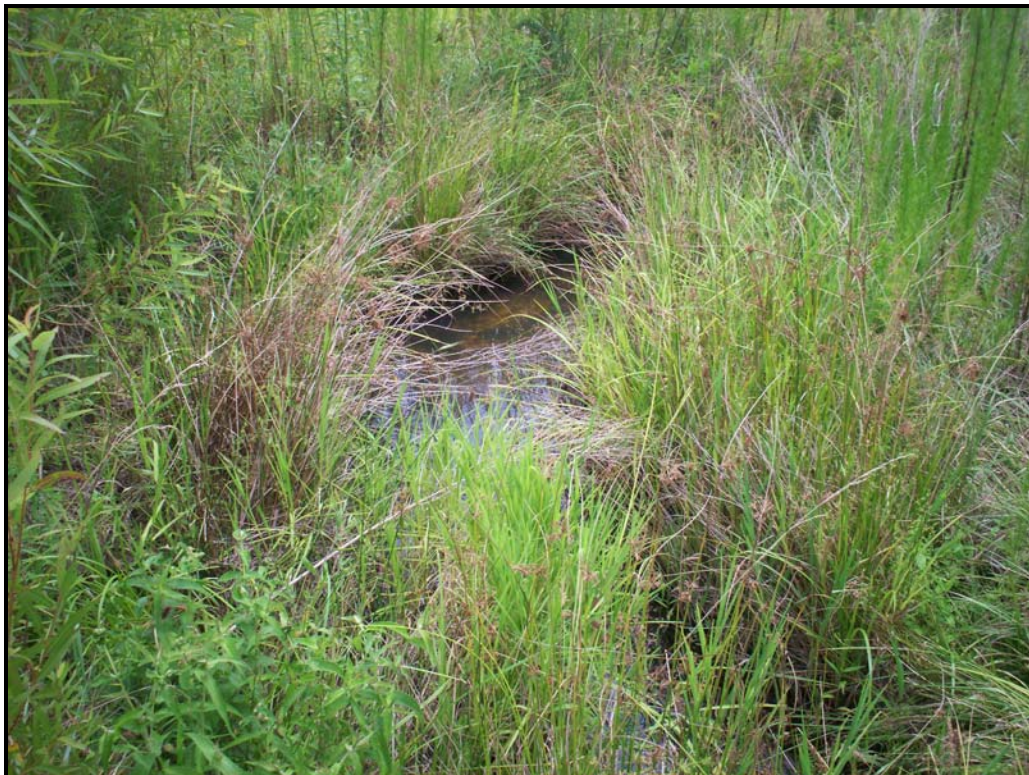
Photo 8. Grade control structure with well vegetated banks at STA 3+40 - looking downstream.
