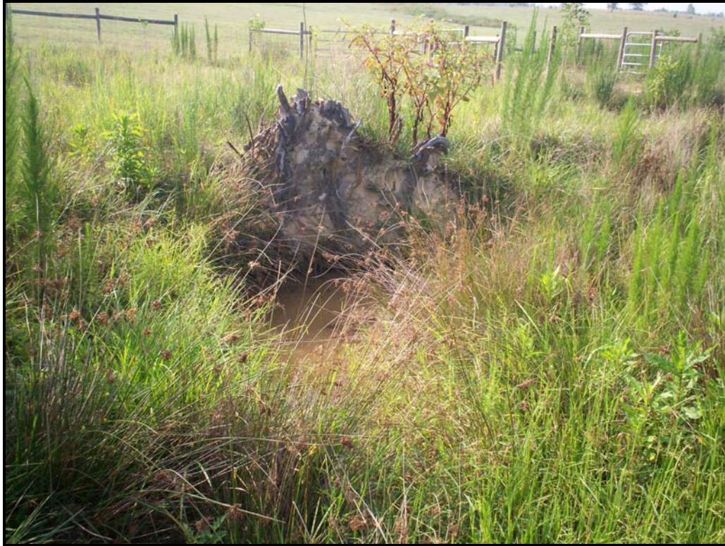
Photo 5. Root wad on left bank at STA 21+00 - looking downstream.
