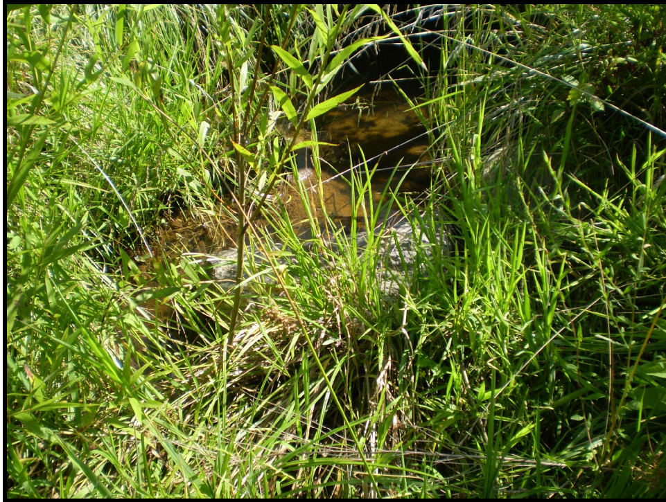
SPA 2 – Rocks displaced at cross weir, UT1 Sta. 8+65.
