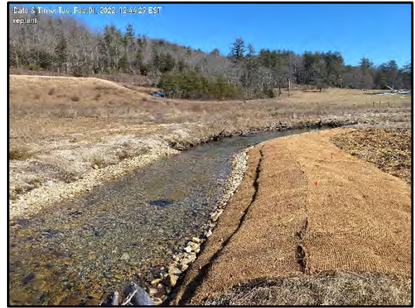
3.40 Repaired right bank using double soil lifts at XS 3 WFFBR, 2/1/2022
