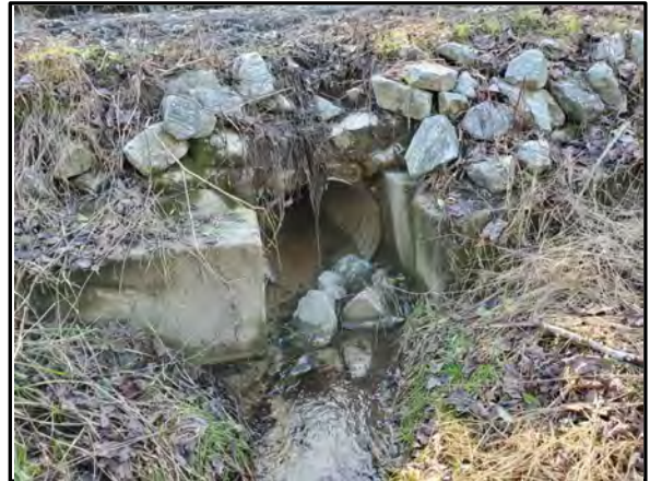
3.32 UT2 Culvert looking upstream, 1/20/2023
