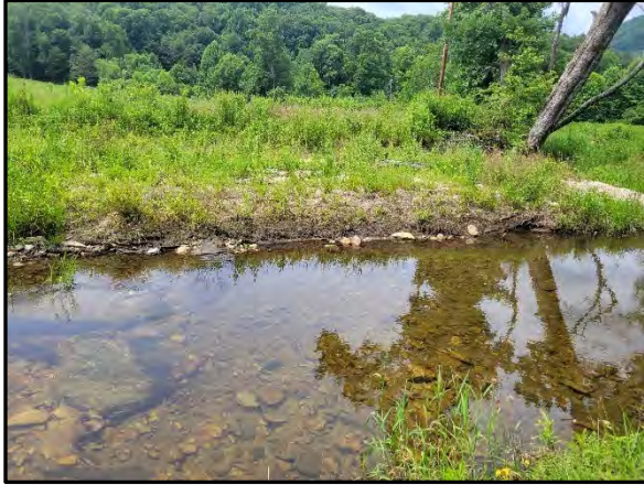
3.43 Bank erosion from STA 10+00 to STA 10+40 WFFBR, 8/15/2022
