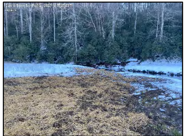
3.42 Repaired left floodplain scour at STA 28 +00 WFFBR, 2/1/2022
