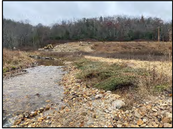
3.50 Bank erosion repair using sod mats from STA 16+10 to STA 16+75 WFFBR, 11/11/2022
