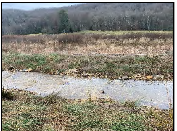
3.48 Bank erosion repair using sod mats from STA 13+90 to STA 14+50 WFFBR, 11/11/2022
