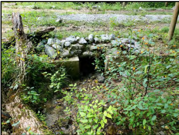
3.29 UT2A Culvert looking downstream, 8/15/2022
