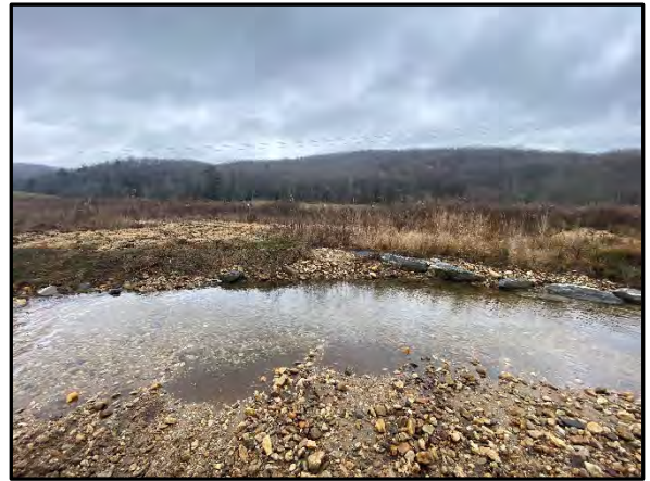
3.46 Bank erosion repair using sod mats from STA 10+70 to STA 11+25 WFFBR, 11/11/2022
