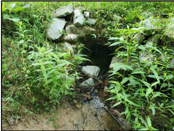
3.31 UT2 Culvert looking downstream, 8/15/2022
