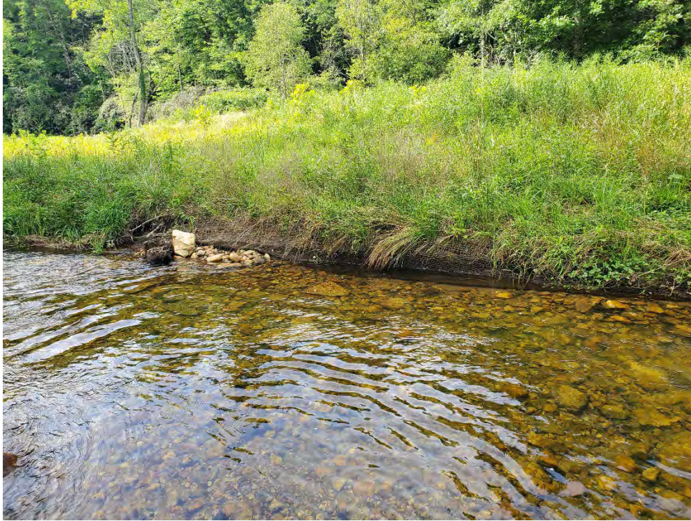
P11: Looking downstream at toe erosion on right bank near Station 25+50
