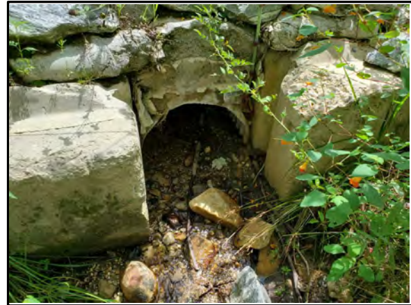
3.28 UT1 Culvert looking upstream, 8/15/2022
