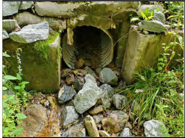
3.30 UT2A Culvert looking upstream, 8/15/2022
