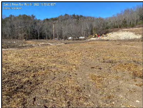
3.41 Expanded left floodplain near STA 17+00 WFFBR, 2/1/2022
