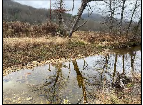
3.44 Bank erosion repair using sod mats from STA 10+00 to STA 10+40 WFFBR, 11/11/2022
