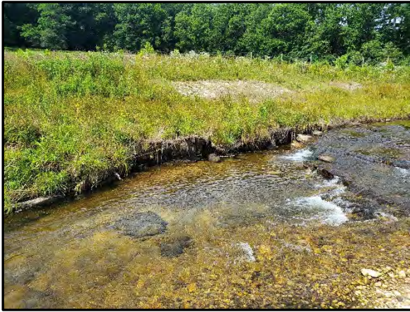
3.51 Toe erosion between STA 22+35 and STA 22+95 WFFBR, 8/15/2022
