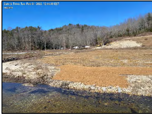
3.39 Repaired left bank near XS 3 WFFBR, 2/1/2022
