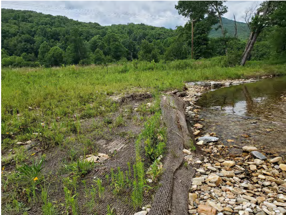
P2: Looking upstream at eroded right bank near Station 11+00
