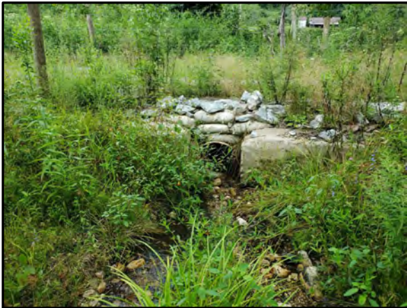
3.27 UT1 Culvert looking downstream, 8/15/2022
