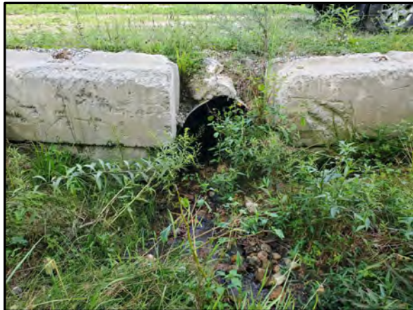
3.33 UT4 Culvert looking downstream, 8/15/2022
