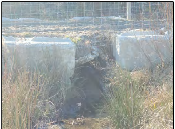
3.34 UT4 Culvert looking upstream, 1/20/2023
