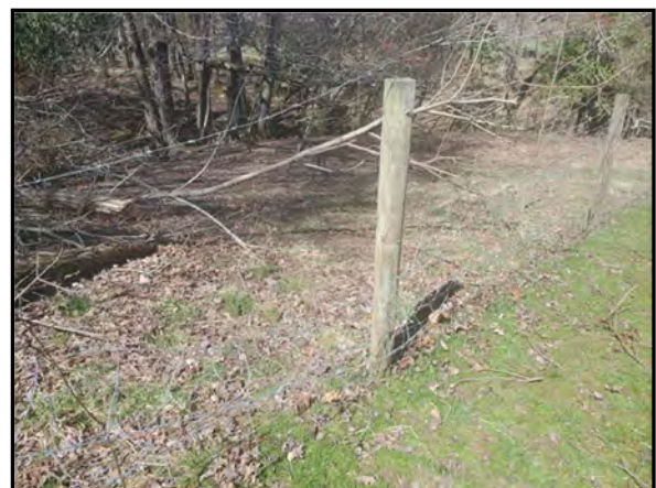
3.36 Downed fence line along UT4: 3/30/2023
