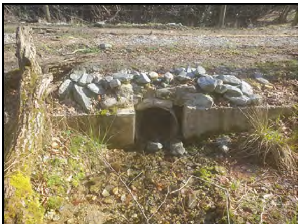
3.29 UT2A Culvert looking downstream, 3/30/2023
