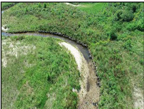
3.23 Aerial overview of UT3 and West Fork French Broad River confluence: 8/24/2023
