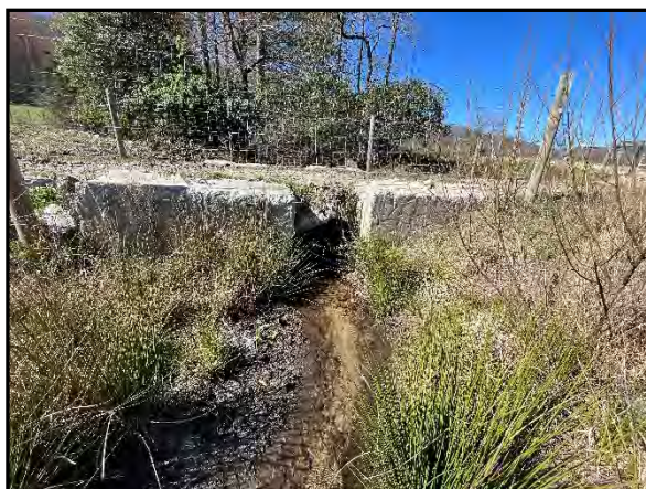
3.35 UT4 Culvert Crossing looking upstream: 3/30/2023
