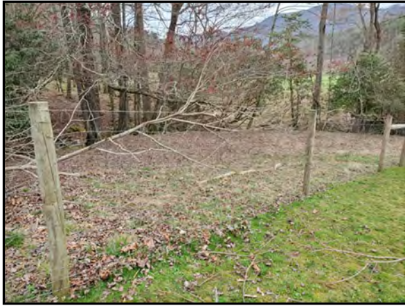
3.37 Repaired fence line along UT4: 3/30/2023
