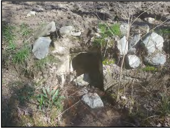
3.31 UT2 Culvert looking downstream: 3/30/2023
