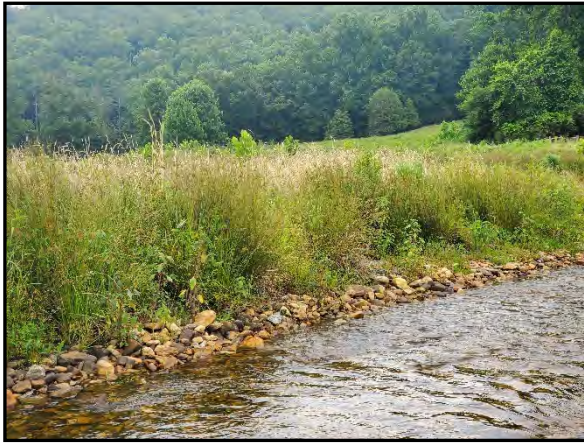
3.45 Juncus sod mat repair at STA 16+50 WFFBR: 6/30/2023
