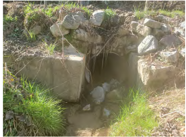
3.32 UT2 Culvert looking upstream: 3/30/2023
