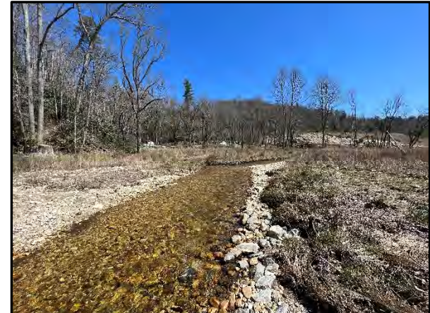
3.42 Repaired area near STA 10+00 WFFBR: 3/30/2023
