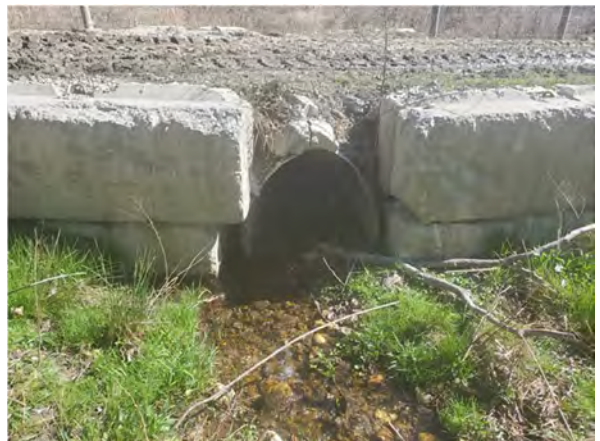
3.34 UT4 Culvert looking downstream: 3/30/2023
