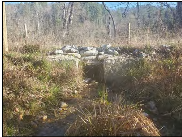
3.27 UT1 Culvert looking downstream: 3/30/2023
