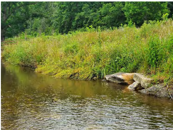
3.47 Juncus sod mat repair at STA 22+35 6/30/2023
