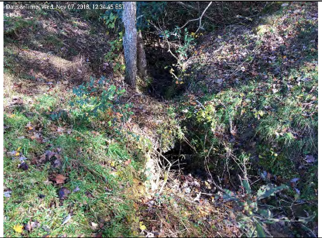
Large headcut on UT 4a near confluence with UT 4
