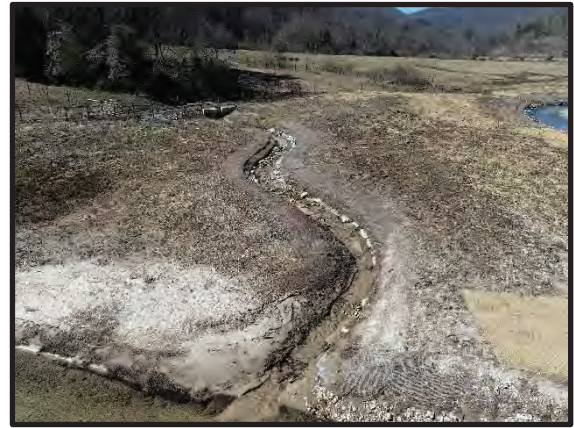
6.24 Aerial overview of UT4, looking upstream
