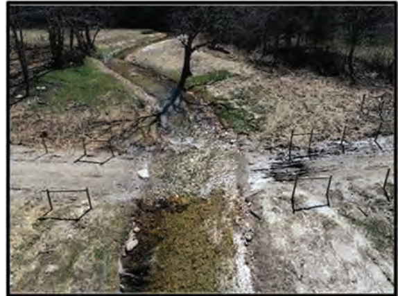
6.26 Downstream view of ford crossing on West Fork French Broad River
