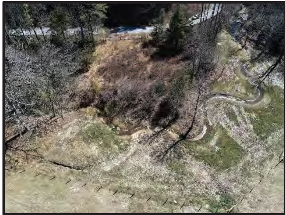
6.27 Aerial overview of UT 7, looking downstream
