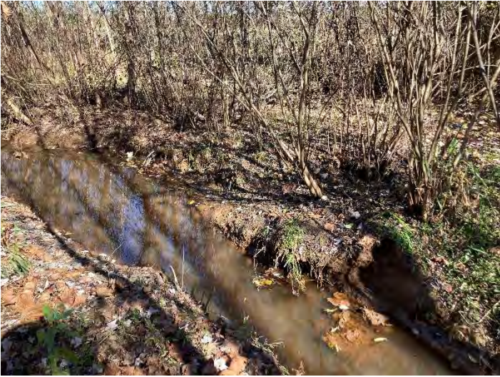
HC1 Reach 2, station 116+15 – Bank scour (11/8/2022)
