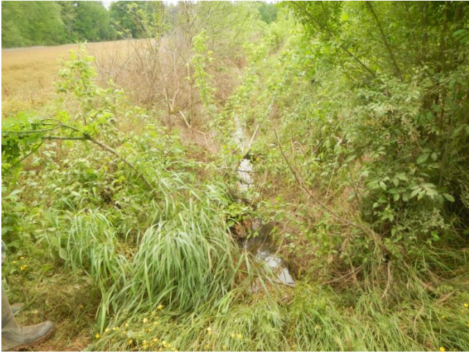
Looking US on culvert (5-8-2013)
