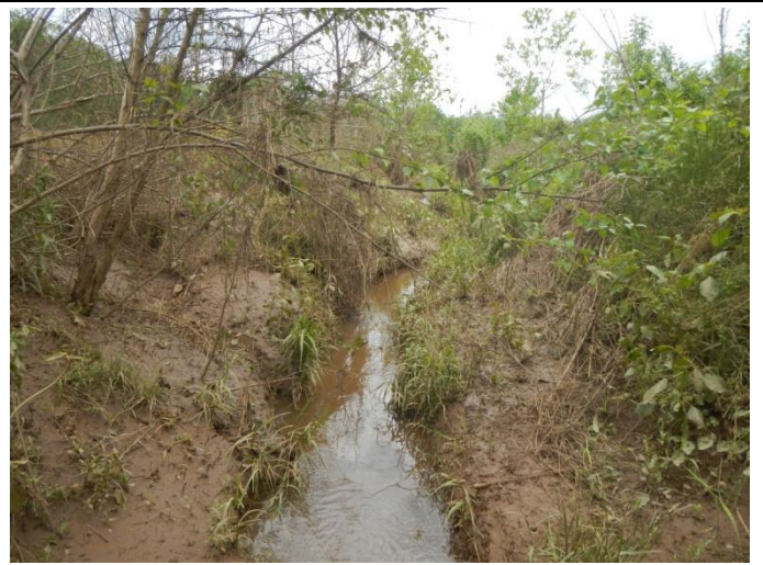
Upstream from culvert (5-8-2013)
