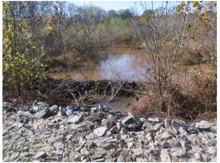
Re-built Beaver Dam above Culvert (11/5/2020)
