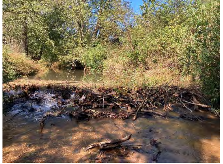
Dam outside of project on Howard's Creek; downstream of confluence (11/10/2021)
