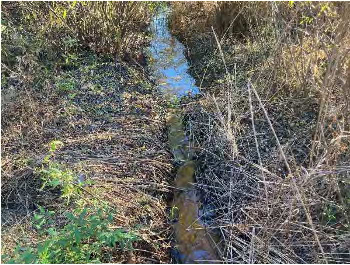
Aggradation on HC2; extends from station 205+50 to station 207+08 (11/10/2020)
