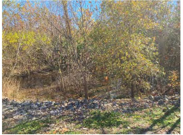
Floodplain inundation from removed beaver dam at station 116+00 (10/18/2021)
