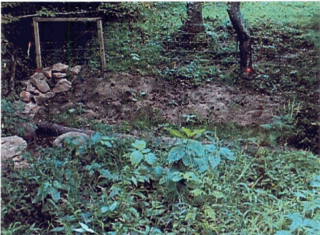
Top photo shows condition of a site that livestock were using to water and cross the stream. Bottom photo shows the same site after coir logs were used to define the channel and the banks were filled and sloped up to the logs. The site was seeded and protected with erosion control blankets. Trees were planted and the stream fenced.
