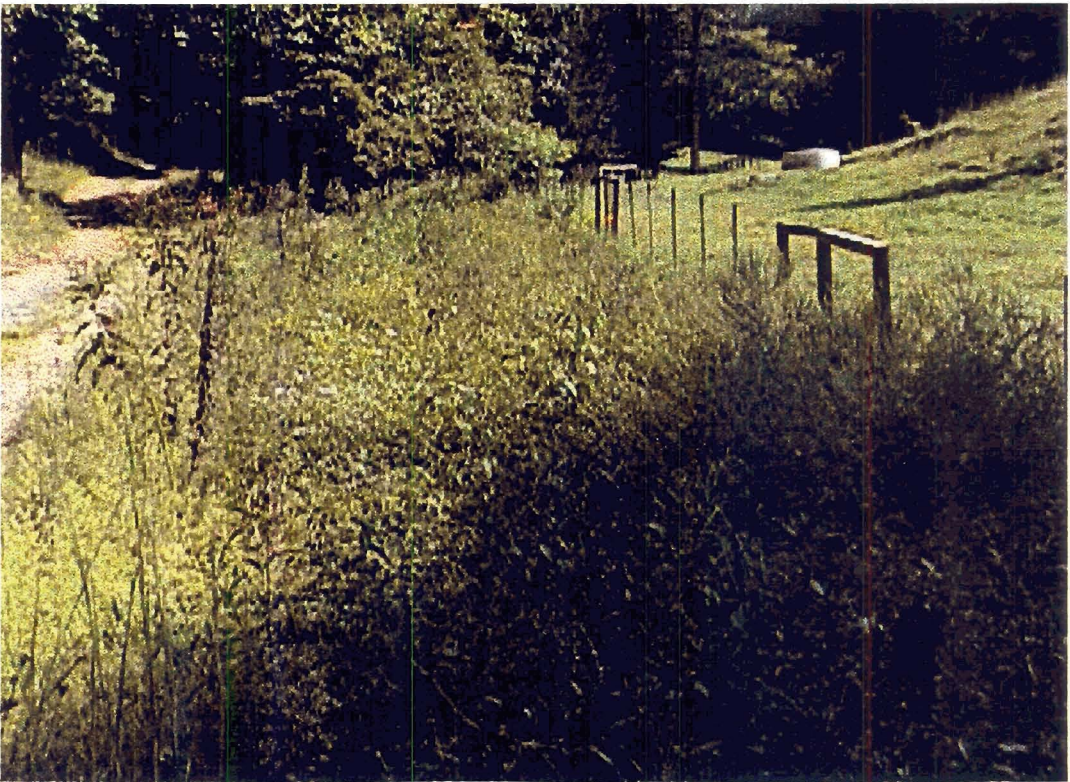
Top photo is along the lower, unnamed tributary looking up stream from the bottom of the reach. Bottom photo is the same site after construction. Vegetation has grown thick on the banks. Livestock were fenced out of this site and one of the water tanks installed at this site can be seen in the background. A covey of quail was flushed at this site when taking this photo.
