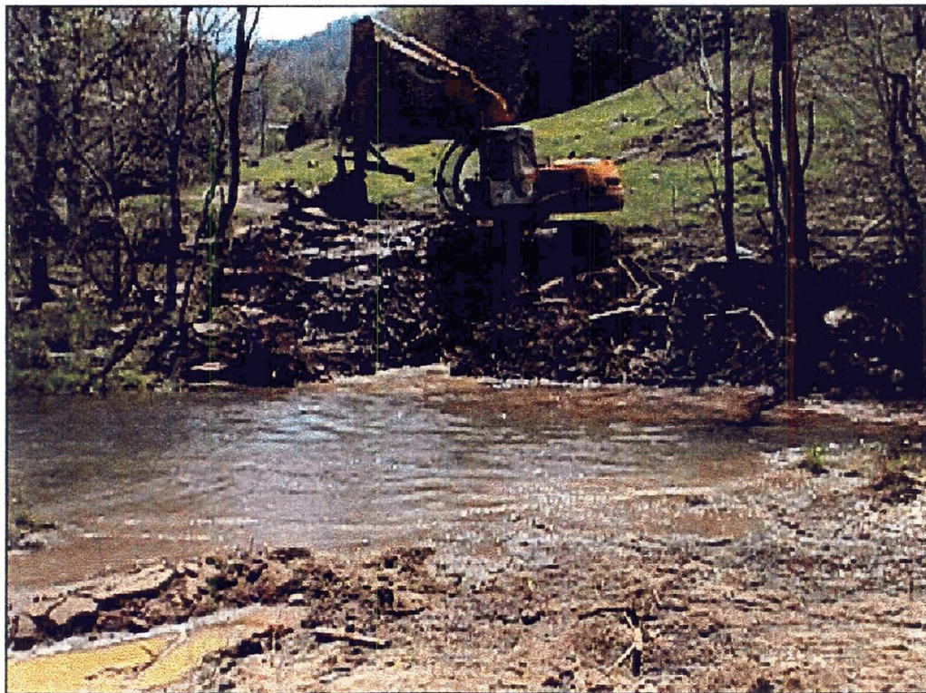
Big bend below driveway bridge. Top photo shows the existing conditions with erosion and auto parts as stabilizing material. Bottom photo shows removing auto parts and trash and installing root-wads and creating floodplain to match existing bench upstream.
