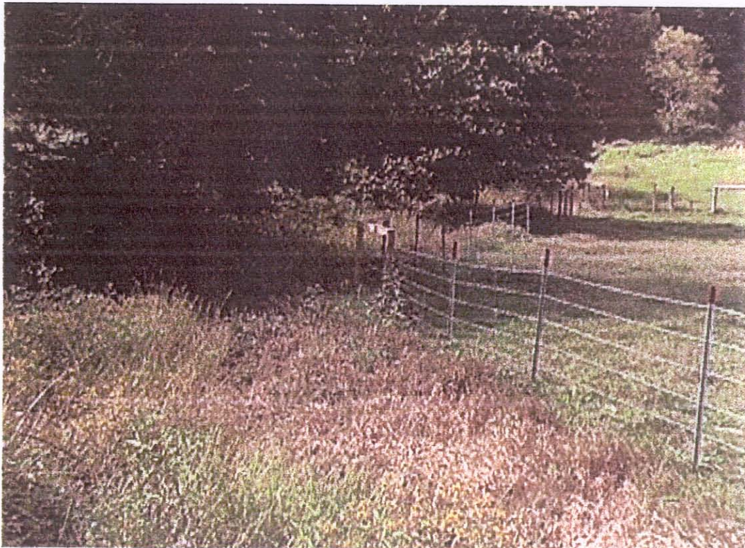
Top photo shows the lower end of the upper, unnamed tributary prior to construction. Bottom photo shows the same site after construction. Banks were sloped and seeded and livestock were fenced out of the site. Prior to construction, the two small unnamed tributaries at this site were major sources of sediment during high water periods.
