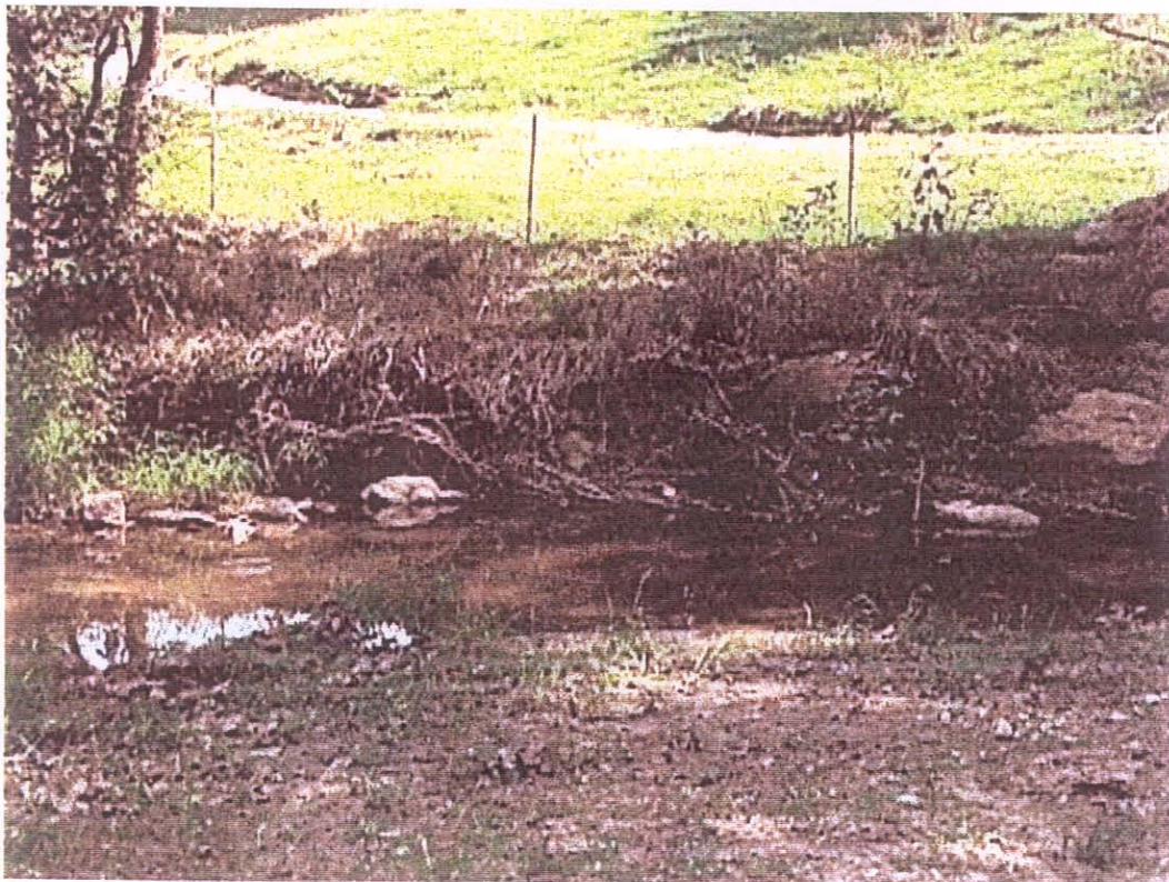
Top photo shows concave side of meander after construction and installation of erosion control material and root-wads. Bottom photo shows flood-plain bench matching the upstream bank with cover crop vegetation, trees and fence 3 months after construction.
