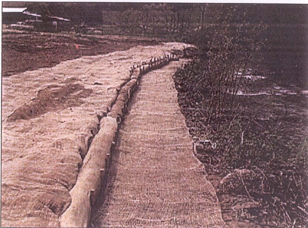
Top photo shows typical condition of stream banks at this site prior to construction. Bottom photo shows typical construction methods used to address vertical bank conditions. Banks are sloped, fertilized, limed, seeded and erosion matting installed. Coir logs are pinned at the bankfull elevation and trees are planted behind this log to provide long-term stability.
