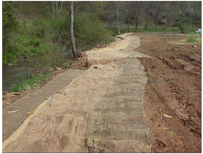
Photo sta. 1, facing upstream from bridge, May 2000.
