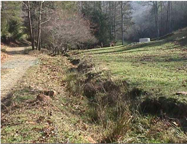
Photo sta. 6, lower tributary facing upstream, November 1999.
