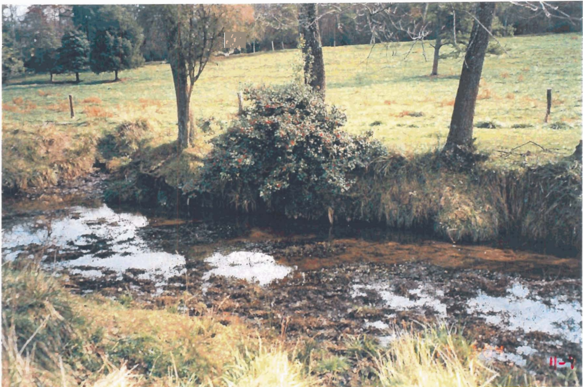
#4 – Bank erosion (typical)
