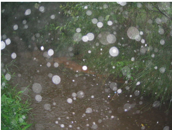
Issue Photo 3. Concentrated sediment laden water cutting through the buffer. Station: End of Area 4.
