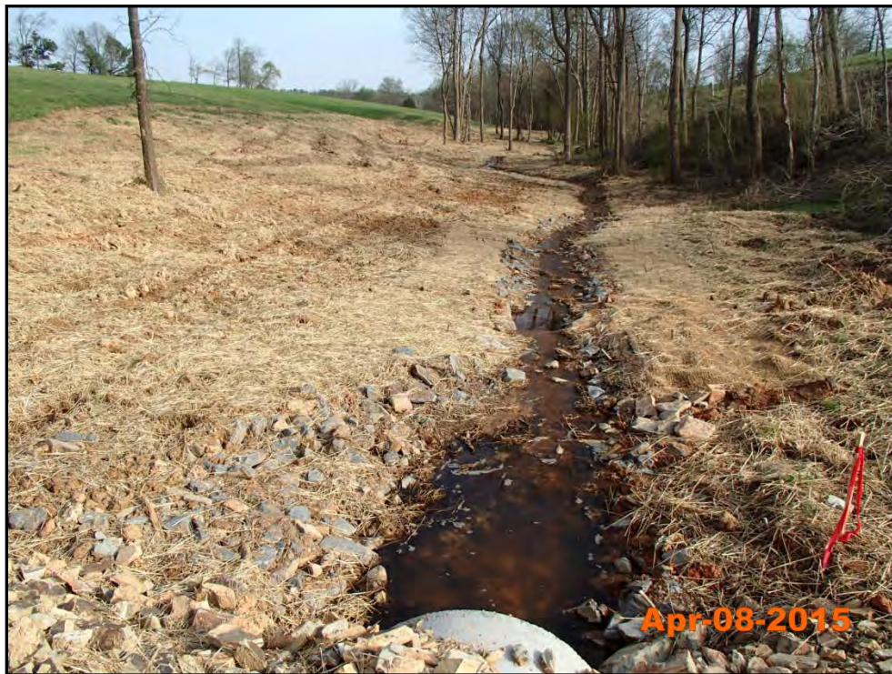
Dale Branch – Permanent Photo Station 8 Station 212+95 - Downstream
