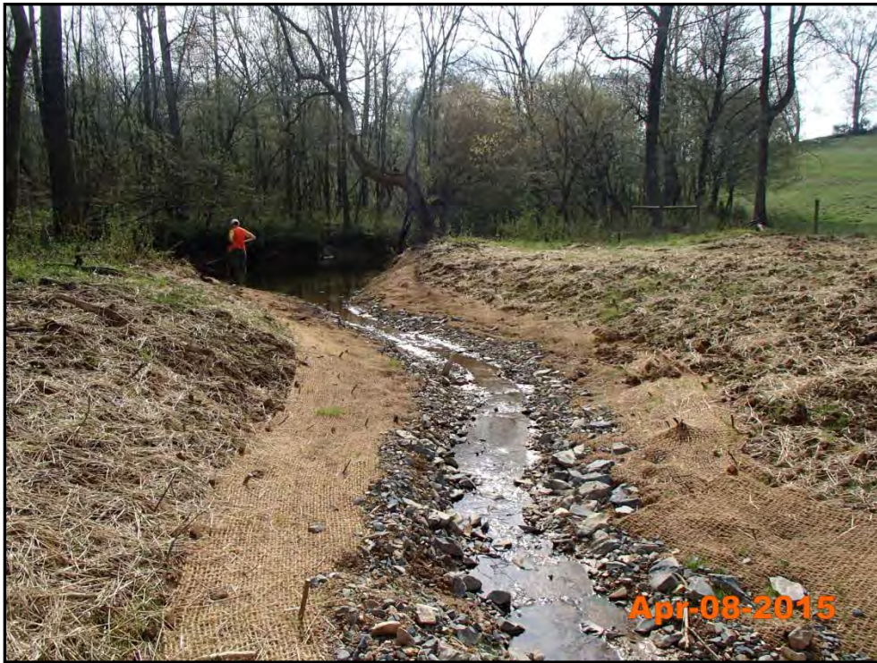
Dale Branch – Permanent Photo Station 12 Station 234+25 – Downstream
