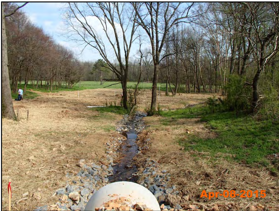
Dale Branch – Permanent Photo Station 11 Station 229+20 – Downstream
