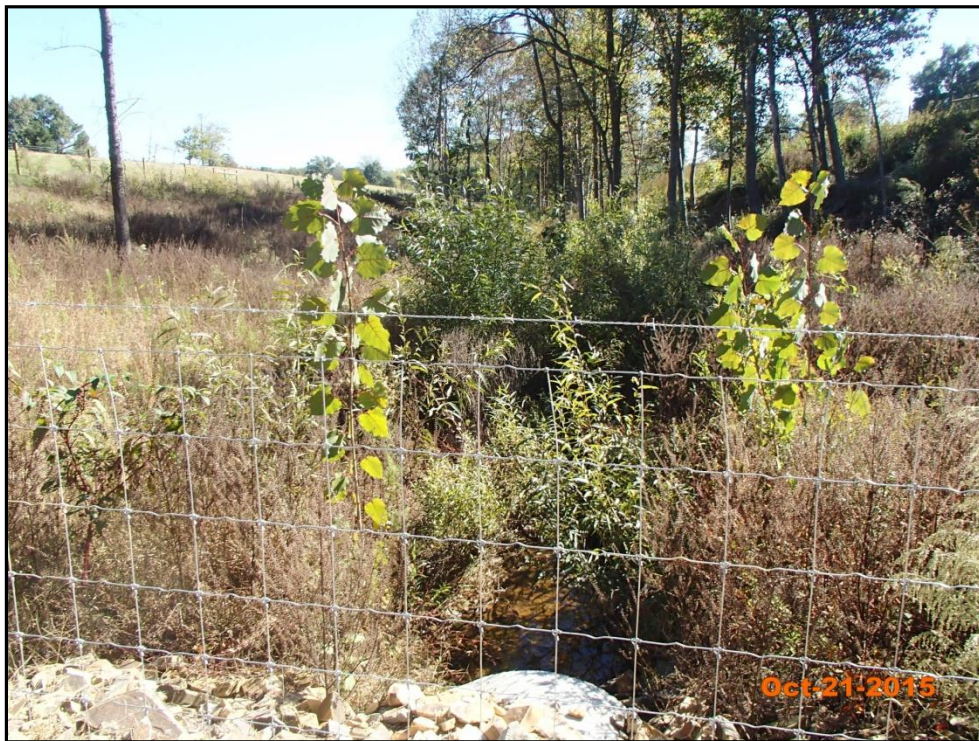
Dale Branch – Permanent Photo Station 8 Station 212+95 - Downstream
