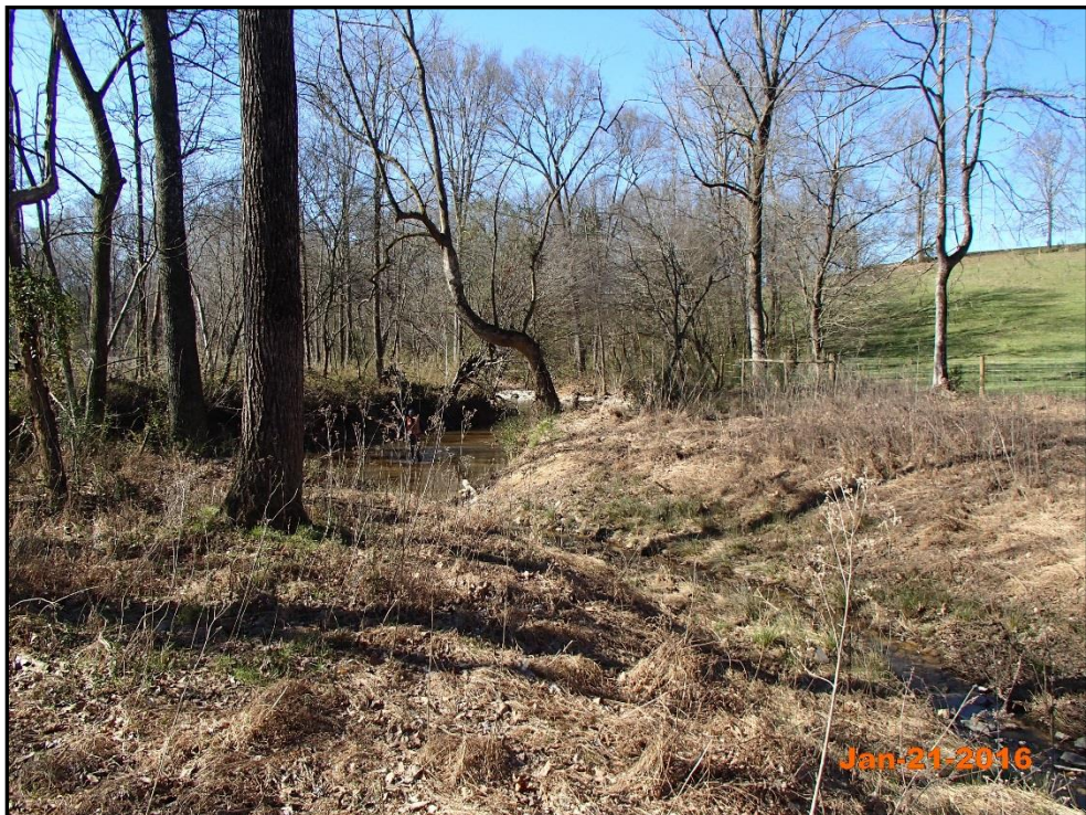
Dale Branch – Permanent Photo Station 12 Station 234+25 – Downstream
