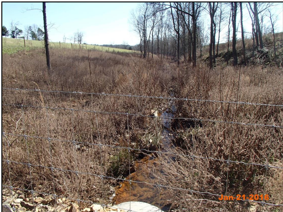
Dale Branch – Permanent Photo Station 8 Station 212+95 - Downstream
