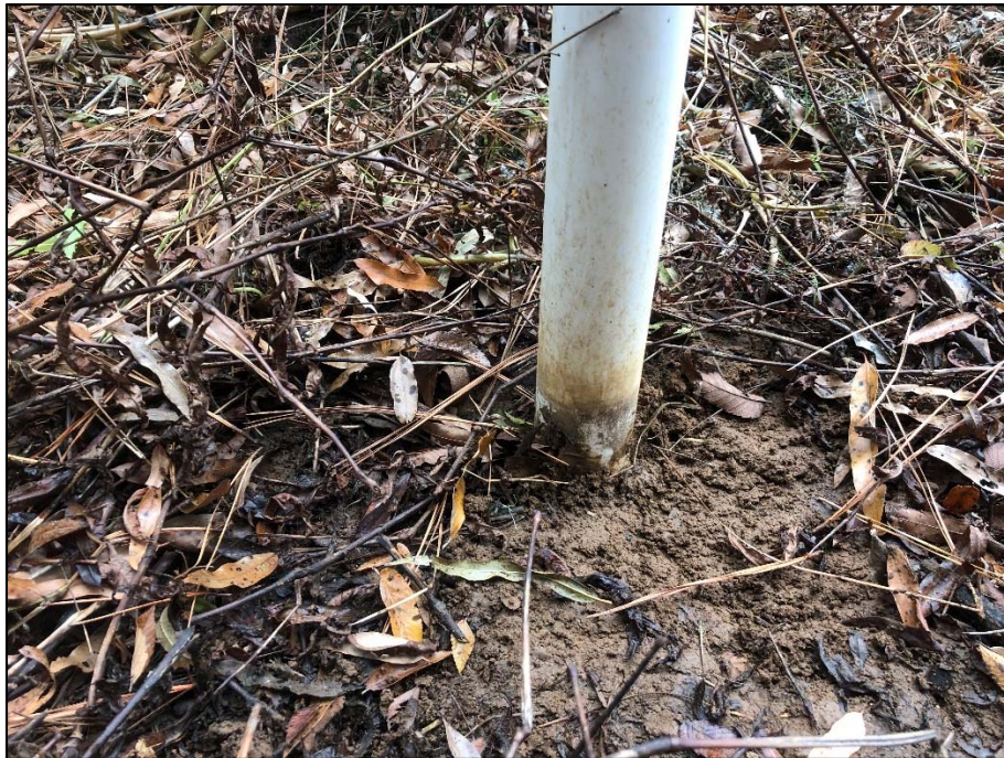
Water stain on FG Dale 1
