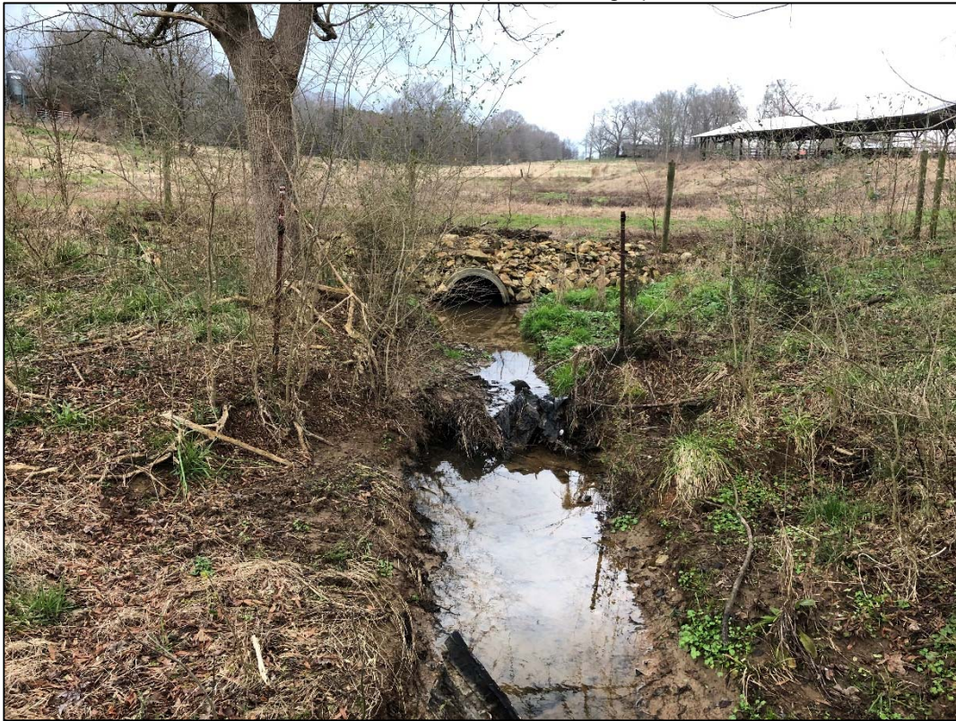
Thompson 1 above old pond looking upstream at new crossing
