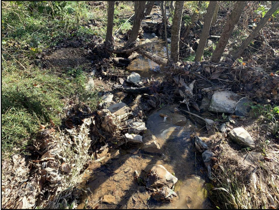
Jerry Branch – Permanent Photo Station 1 Station 300+25 - Downstream
