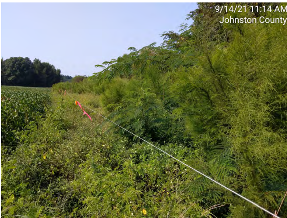
Encroachment (VPA1) R1 Left Floodplain, September 14, 2021 (MY-04)
