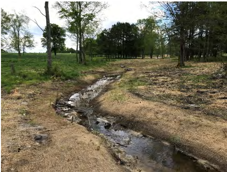
PS-6, R4, facing upstream, Sta 43+50, April 27, 2018 (MY-00)
