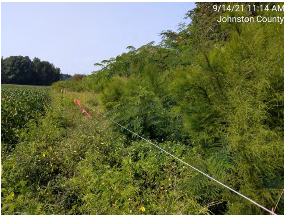
Encroachment (VPA1) R1 Left Floodplain, September 14, 2021 (MY-04)
