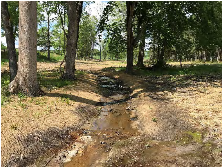
PS-8, R4, facing upstream, Sta 52+00, April 27, 2018 (MY-00)
