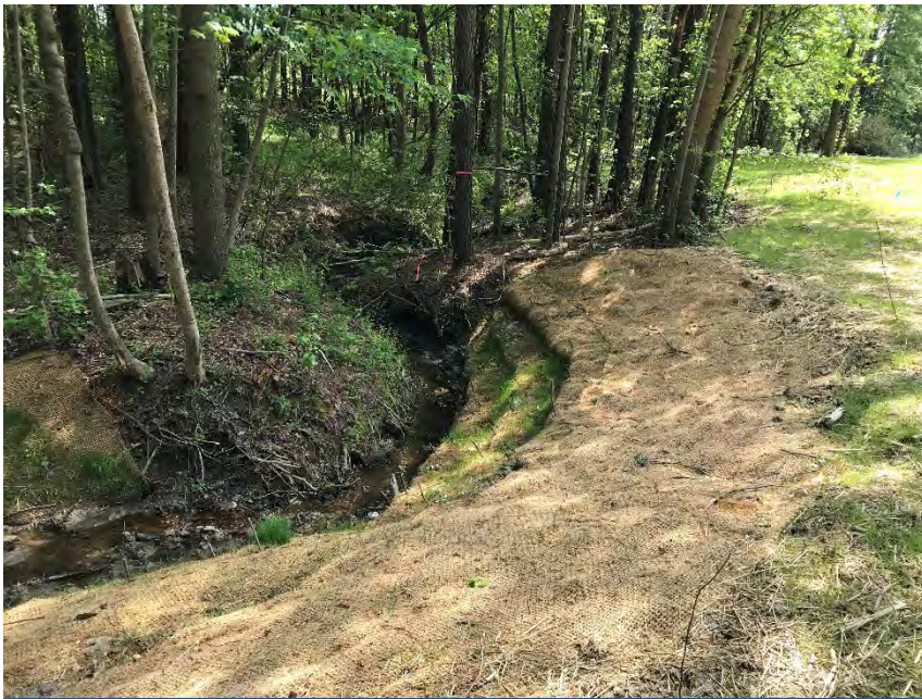
PS-2, R2, facing downstream, Sta 21+50, April 27, 2018 (MY-00)
