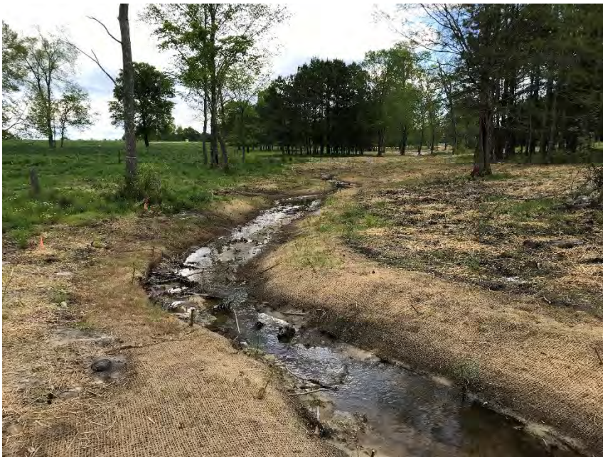
PS-6, R4, facing upstream, Sta 43+50, April 27, 2018 (MY-00)
