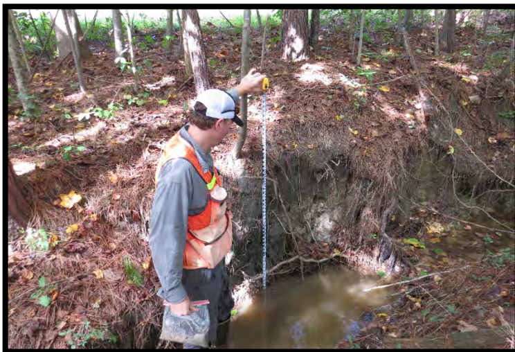
Photo illustrates active bank erosion and headcut migration along upper R2.
