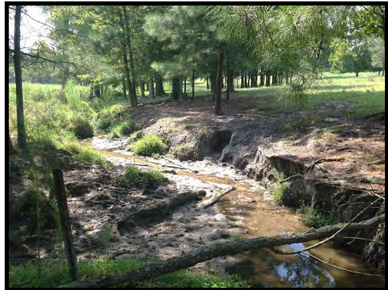
Photo of R4 (upper) looking downstream showing cattle access and severely degraded stream banks.
