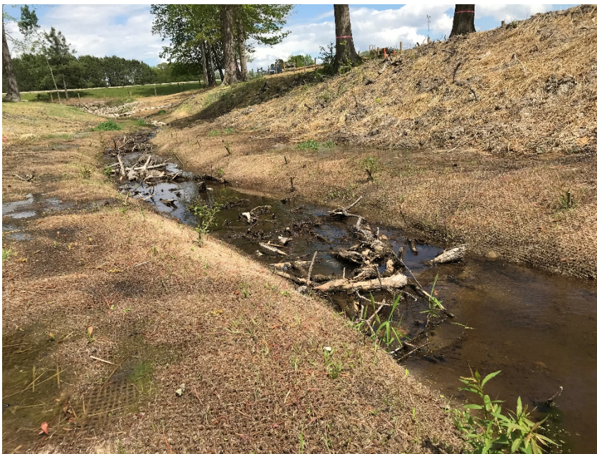
R3, facing upstream, Sta 33+00, April 27, 2018 (MY-00)
