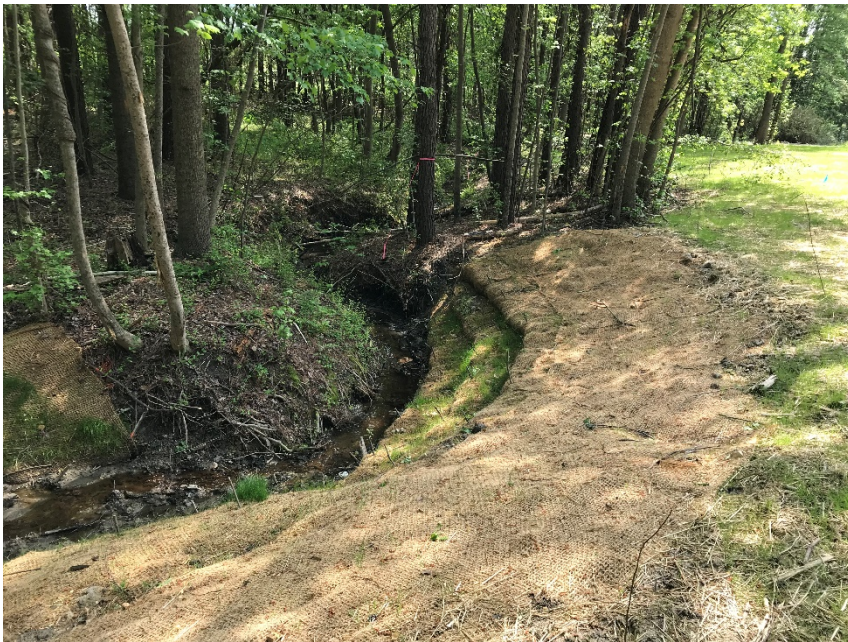
R2, facing downstream, Sta 21+50, April 27, 2018 (MY-00)
