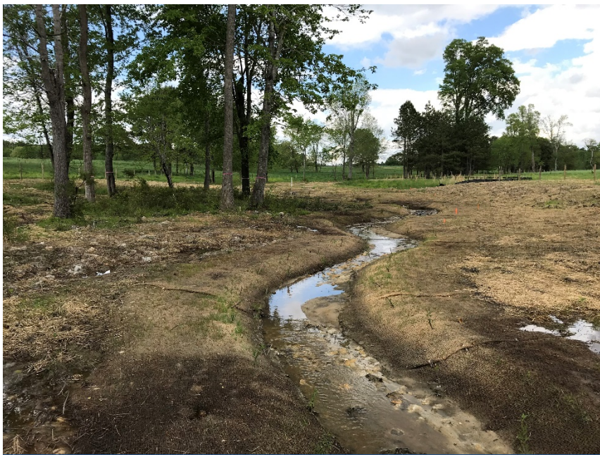
R4, facing upstream, Sta 44+50, April 27, 2018 (MY-00)
