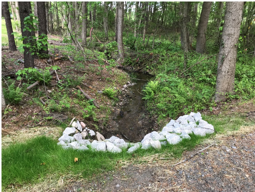
R2, facing upstream at crossing, Sta 23+00, April 27, 2018 (MY-00)
