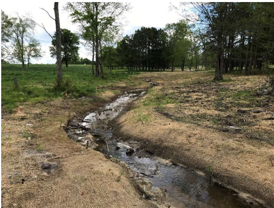
R4, facing upstream, Sta 43+50, April 27, 2018 (MY-00)
