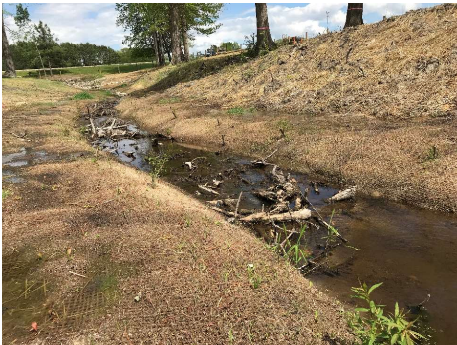
R3, facing upstream, Sta 33+00, April 27, 2018 (MY-00)
