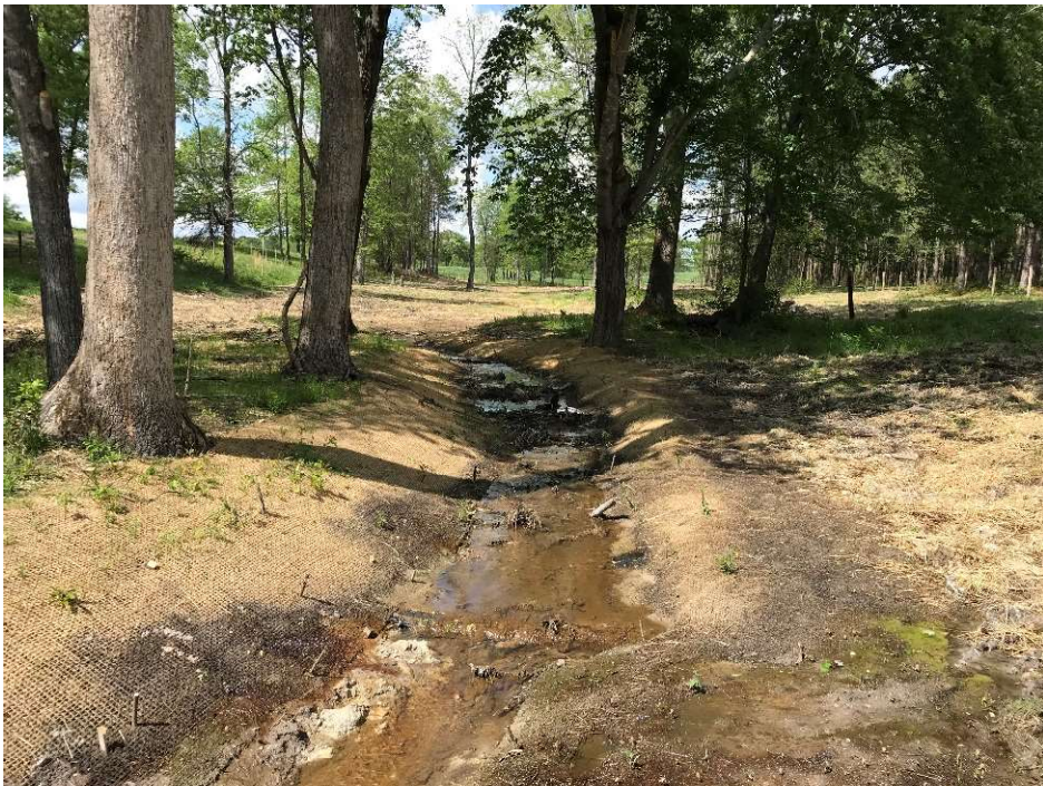
R4, facing upstream, Sta 52+00, April 27, 2018 (MY-00)
