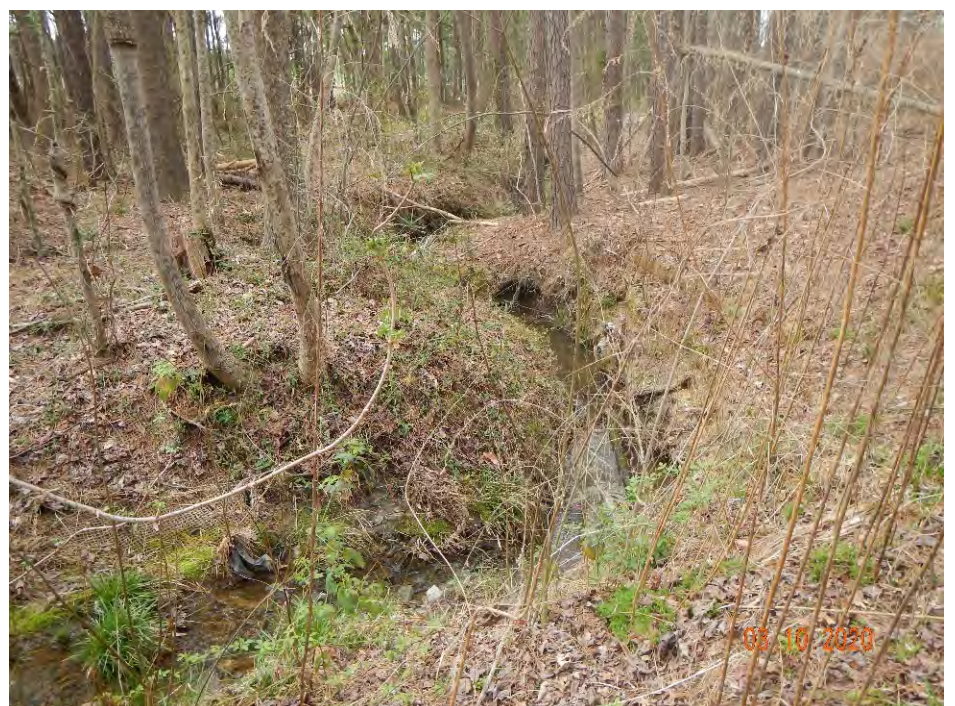
PS-2, R2, facing downstream, Sta 21+50, March 10, 2020 (MY-03)
