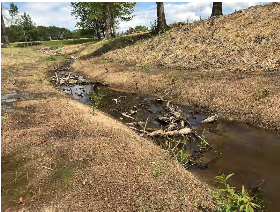
PS-5, R3, facing upstream, Sta 34+00, April 27, 2018 (MY-00)
