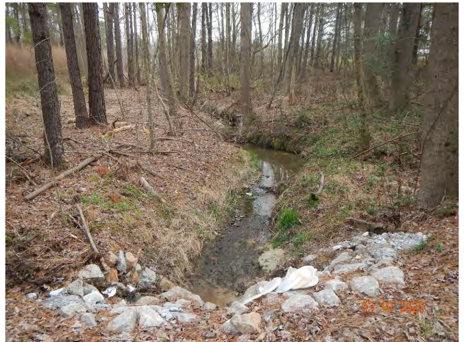
PS-3, R2, facing upstream at crossing, Sta 23+00, March 10, 2020 (MY-03)
