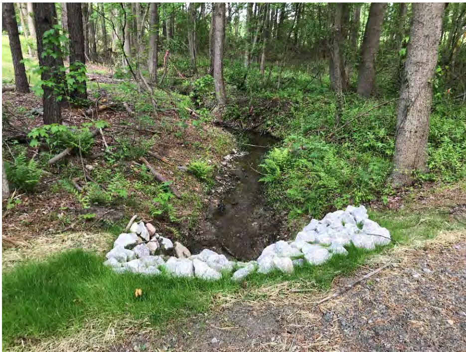
PS-3, R2, facing upstream at crossing, Sta 23+00, April 27, 2018 (MY-00)
