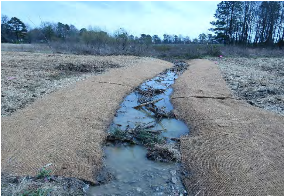
PS-1, R1, facing upstream, Sta 20+00, March 29, 2018 (MY-00)
