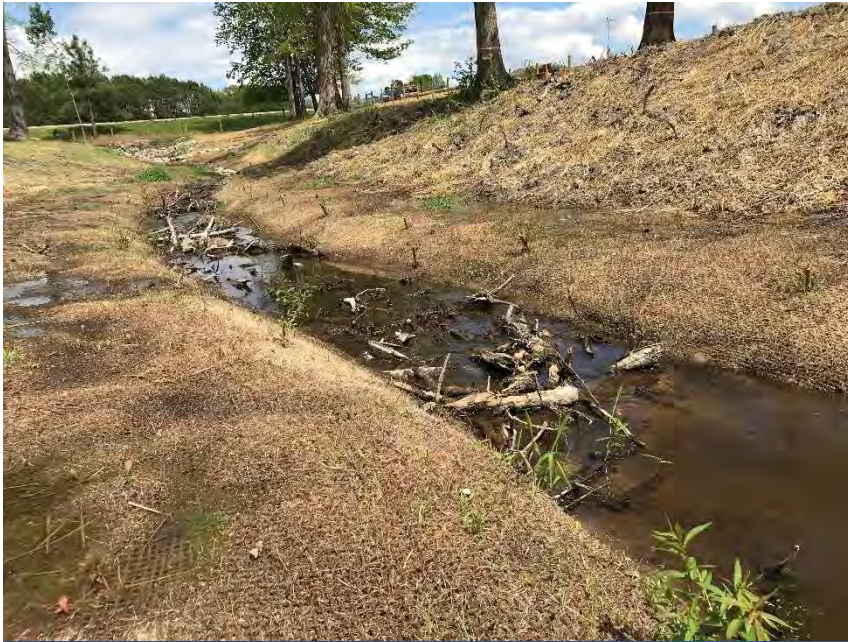
PS-5, R3, facing upstream, Sta 34+00, April 27, 2018 (MY-00)
