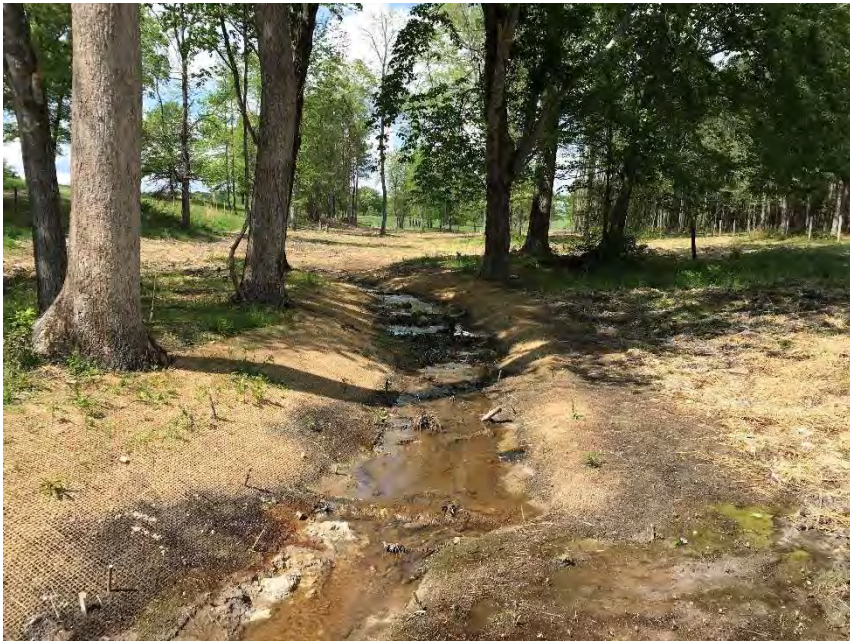
PS-8, R4, facing upstream, Sta 52+00, April 27, 2018 (MY-00)
