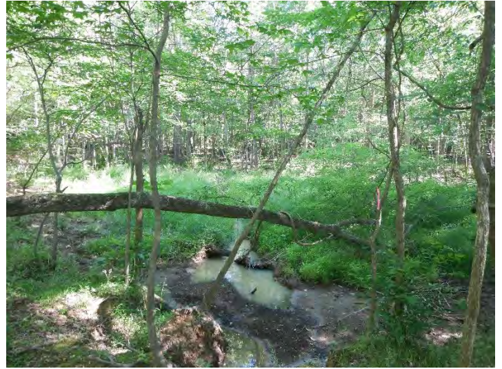
Perry Branch Reach 1 – Breached Impoundment
