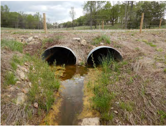
Perry Branch R4 – Looking Upstream (04/14/2022)
