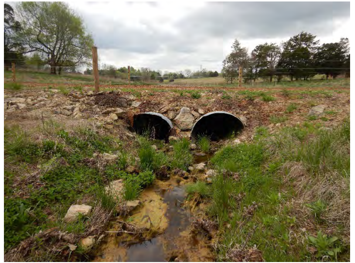
Perry Branch R4 – Looking Downstream (04/14/2022)
