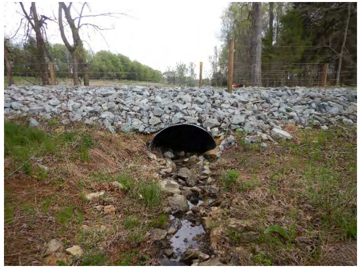
Perry Branch R2 – Looking Downstream (04/14/2022)
