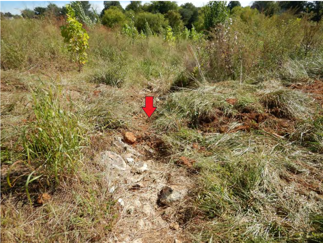
UT1 R1 DS – Repair at end of riffle above rock sill (9/27/2022)
