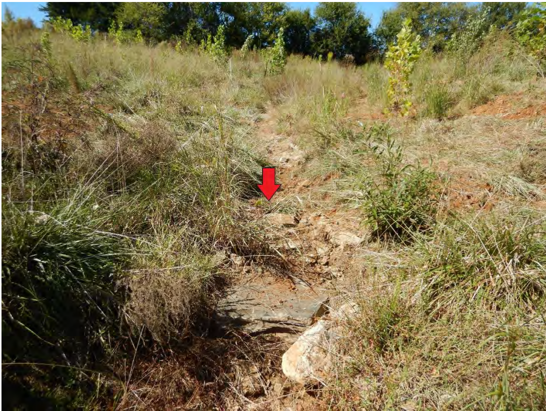
UT1 R1 US – Repair just above rock sill in foreground (9/27/2022)
