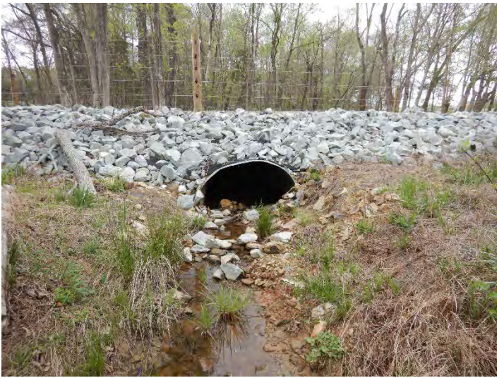
Perry Branch R2 – Looking Upstream (04/14/2022)
