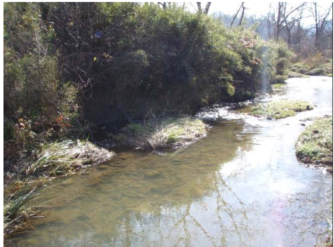
Stream problem area 1, MFC bank sloughing, 25 Nov 2009.
