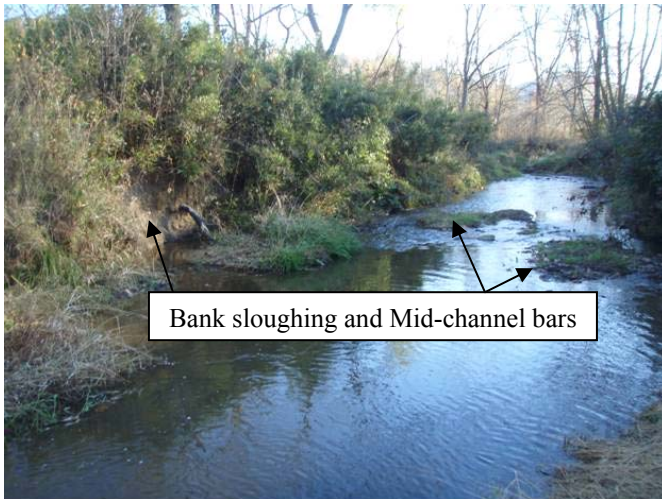
Stream problem area 1, MFC bank sloughing, 4 Dec 2007.
