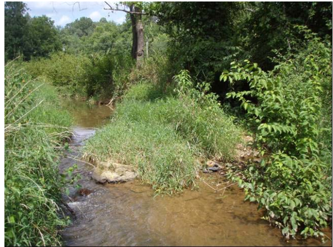
Stream problem area 3, MFC mid channel bar, 25 Nov 2009.
