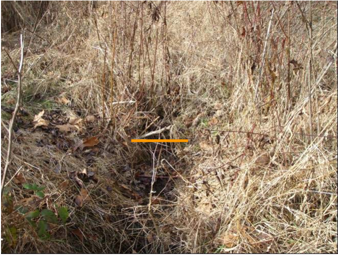
MB cross-section 5, facing downstream, 3 Nov 2009.
